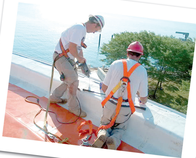
Photo 5 – Custom fabricated, PVC-coated metal is installed to complete the parapet wall detail.
