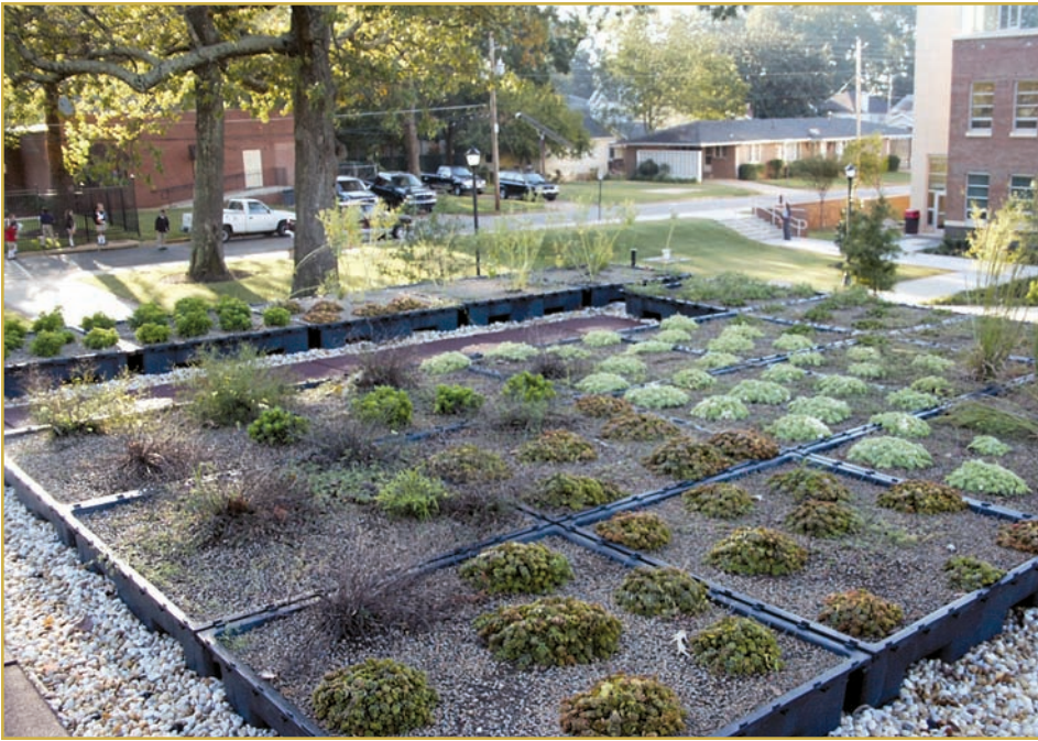
Figure 4 - Jordan N. Carlos Middle School Art Building, Woodward Academy, Atlanta, GA.
