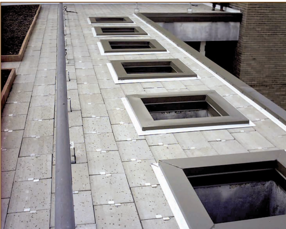
Typical perimeter paver condition.
