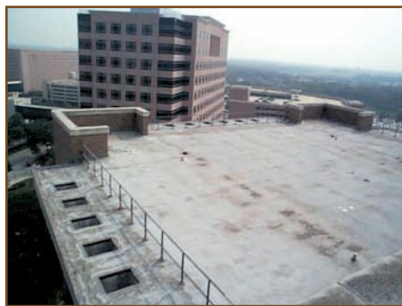
Overview of roof area prior to replacement.
