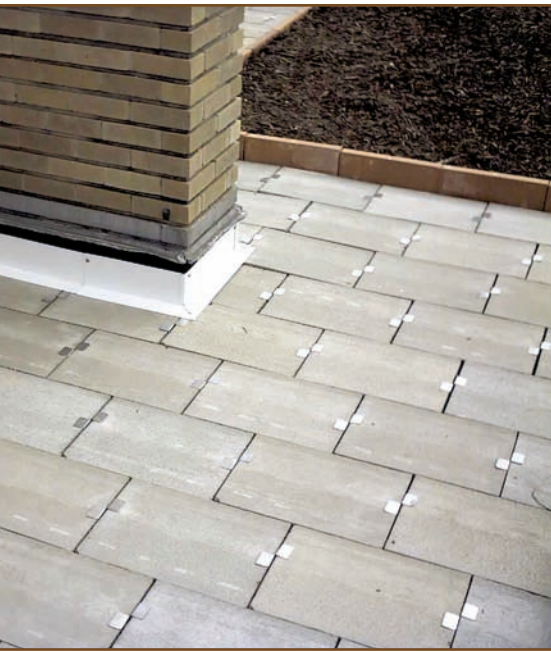
Typical wall flashing.
