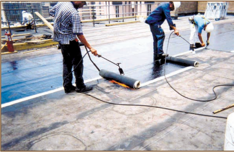
Installation of membrane.
