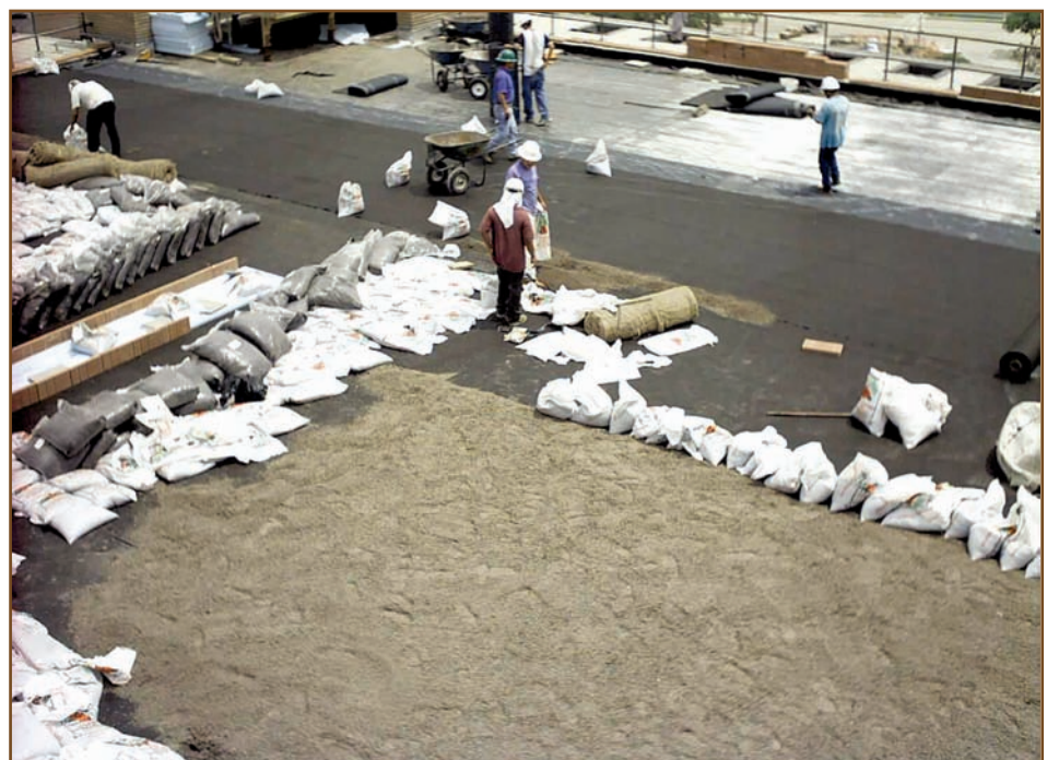
Placement of soil.
