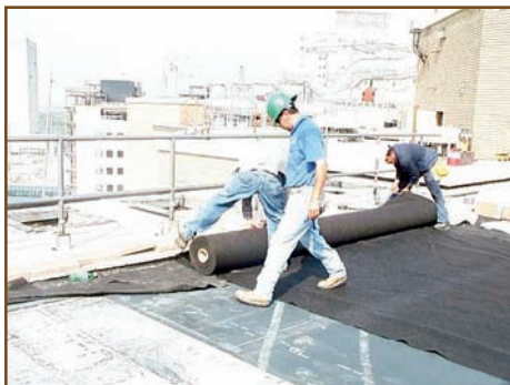
Installation of drain board.
