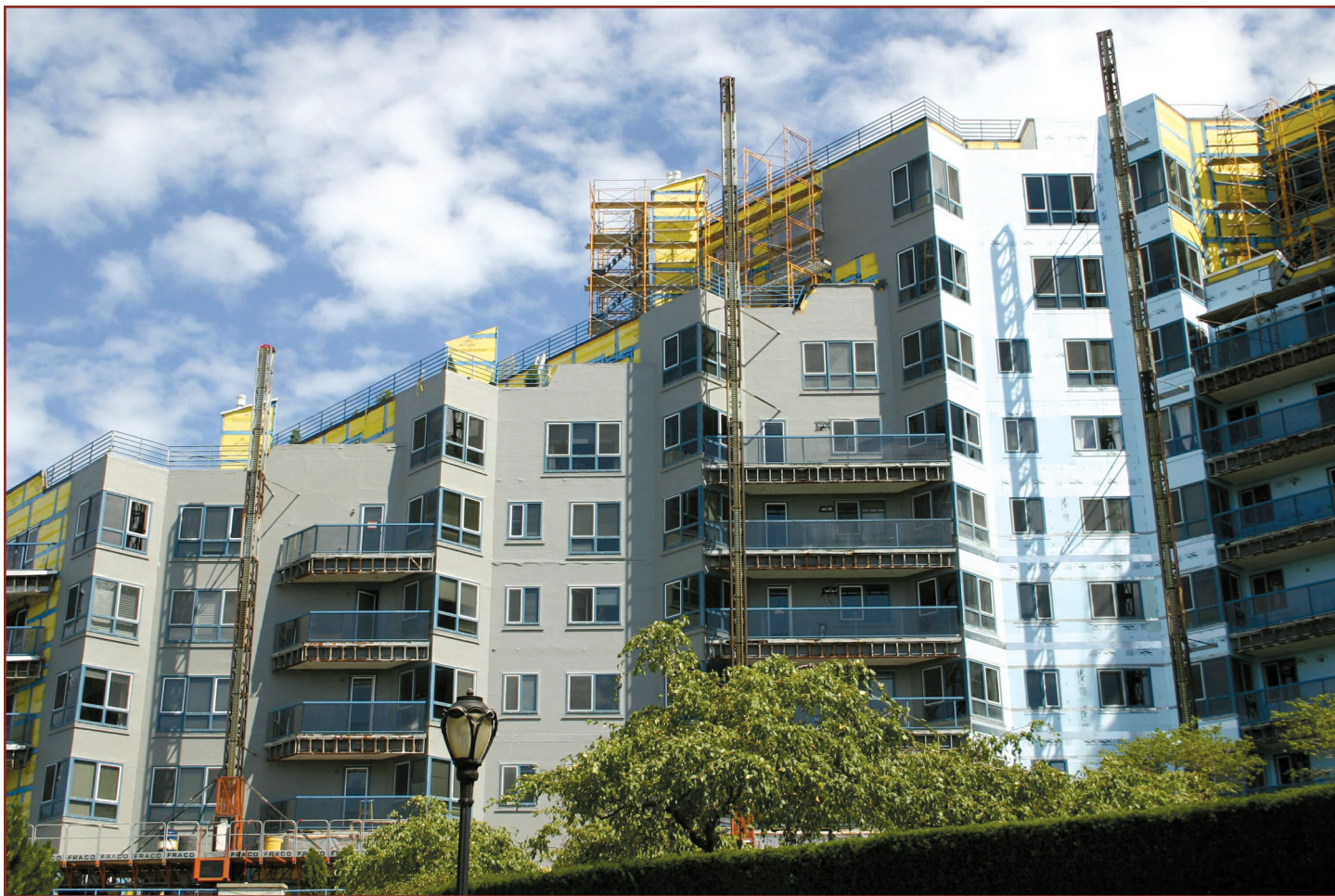
The Marina Bay Tower in Quincy, MA, used Georgia Pacific's DensGlass Gold Sheathing (yellow in photo), Henry's Air-bloc 31 membrane (a liquid emulsion, vapor-permeable air barrier), Dow 1" extruded polystyrene insulation (light blue), and an Alucobond panel system. It is also shown on the cover of this publication.
