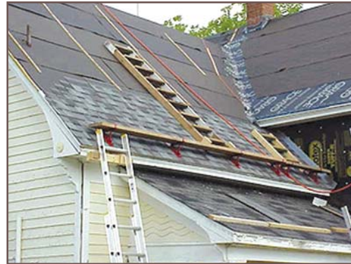
Typical installation of felt and ice dam protection.
