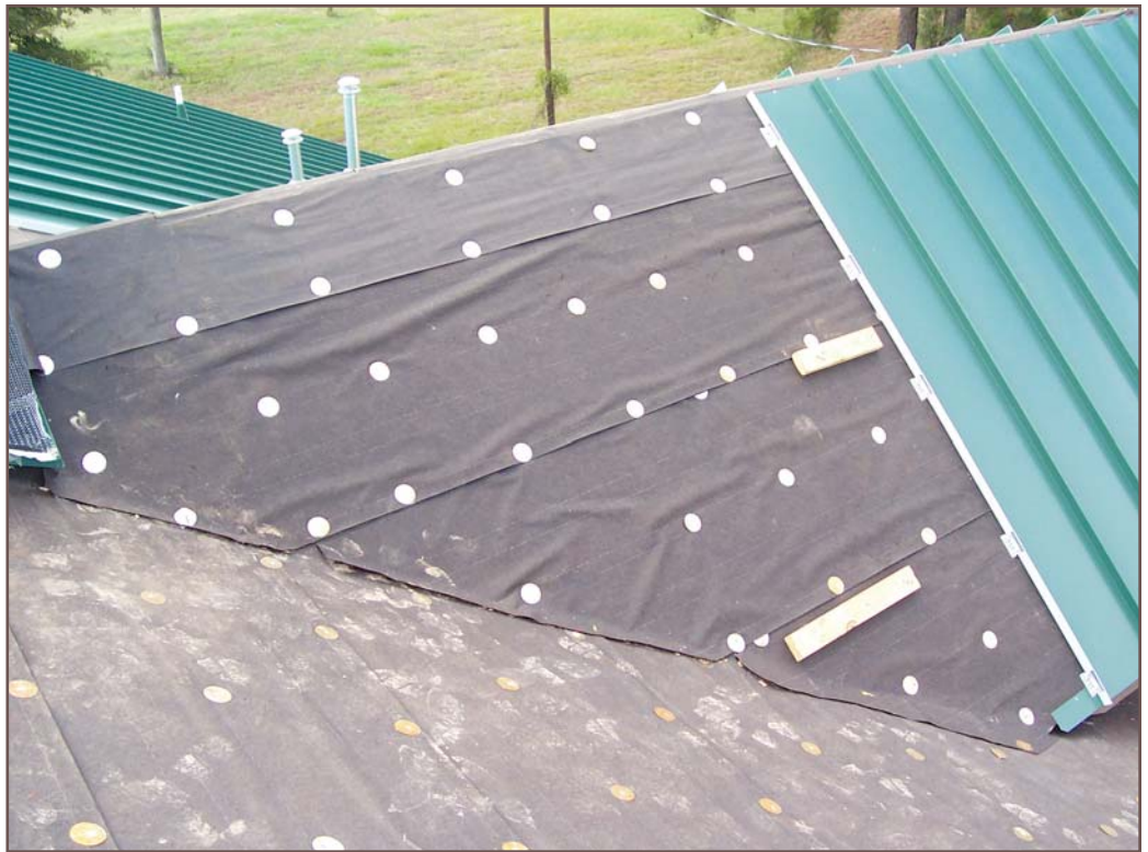
Typical wrinkled organic felt underlayment.
