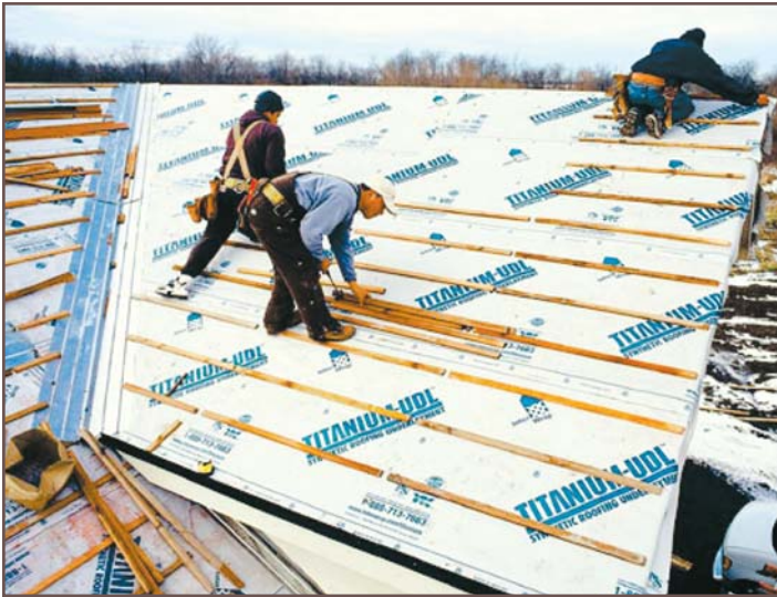
Typical synthetic underlayment installation under tile.
