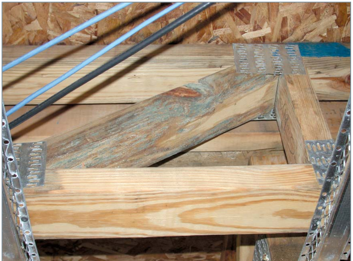
Mold on dimensional lumber.
