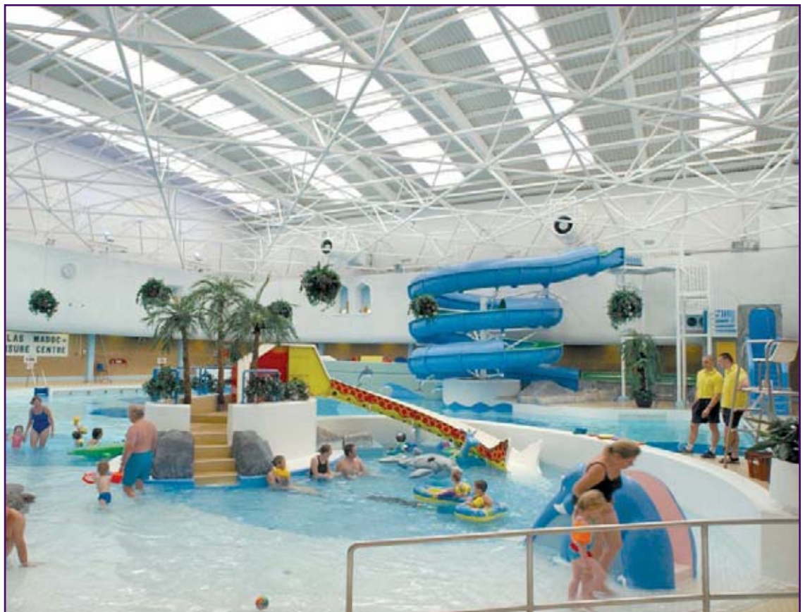
Increasing the skylight area reduces the need for artificial light, cuts the energy requirement of the building, and reduces CO 2 emissions.
