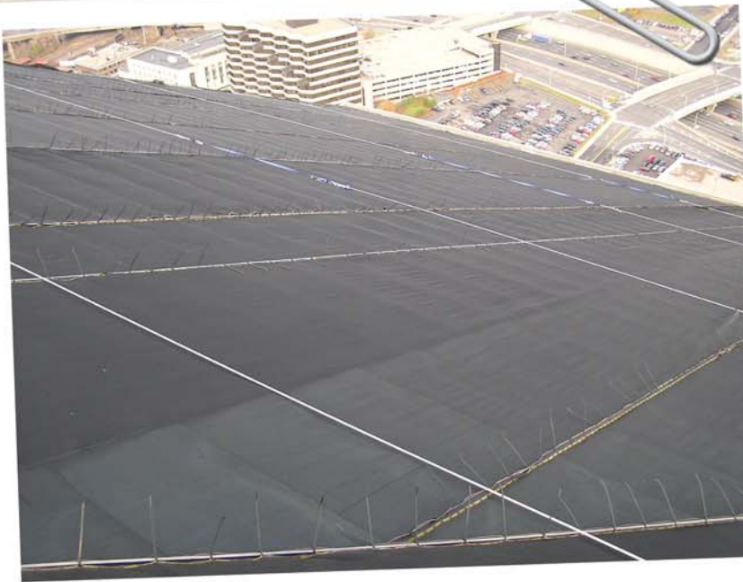
Photo 9: Debris netting on north elevation.
