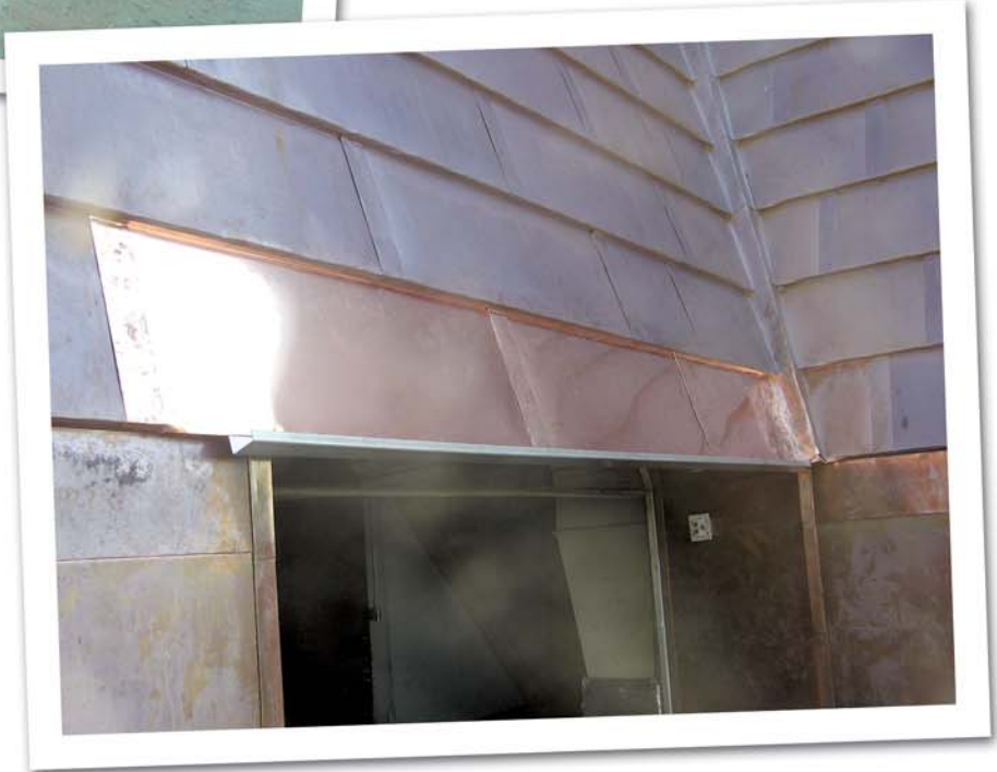
Photo 15: Roll-up door with protective gutter/bumper.
