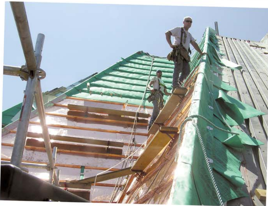
Photo 21: Specialty metal brackets used to provide worker access.
