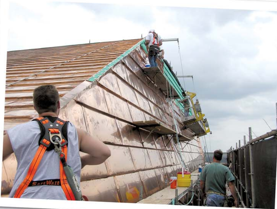
Photo 22: Specialty metal brackets and hanging scaffolds used to provide worker access.
