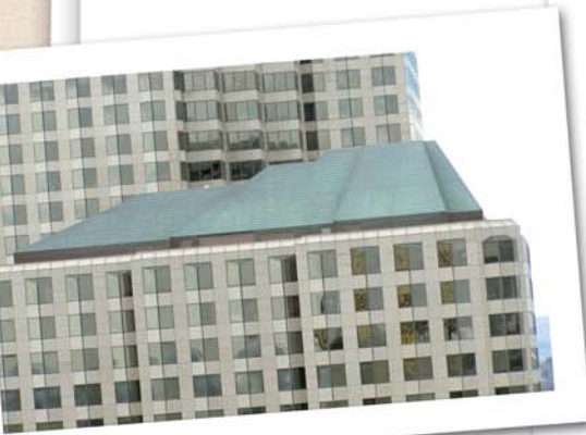
Photo 10: Photo of existing copper roofing.
