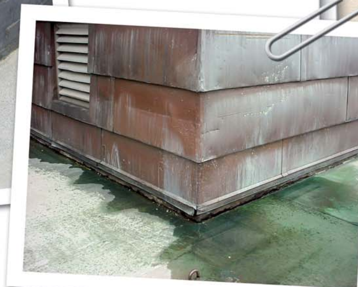
Photos 1 and 2: Damages cause by window-washing rig.
