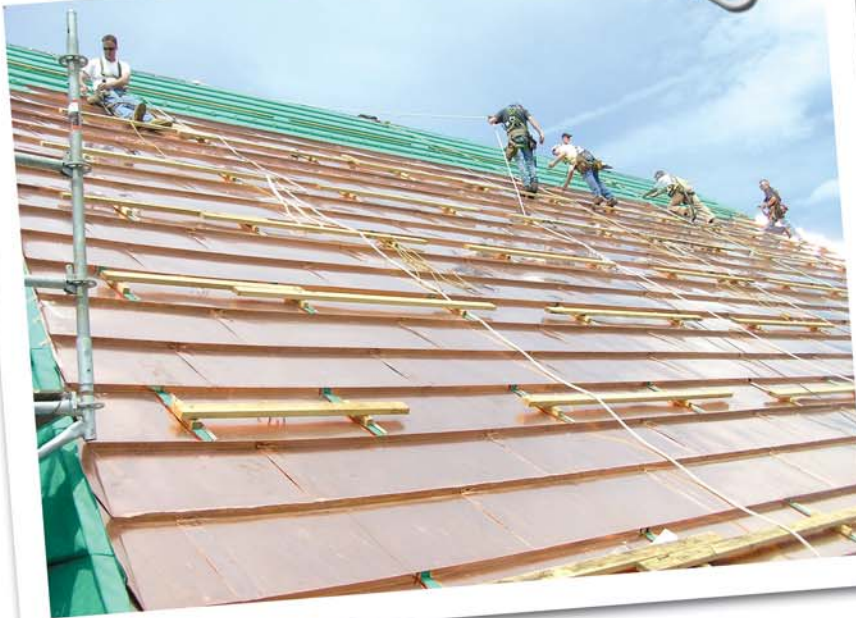
Photo 20: Wood brackets used to provide worker access.
