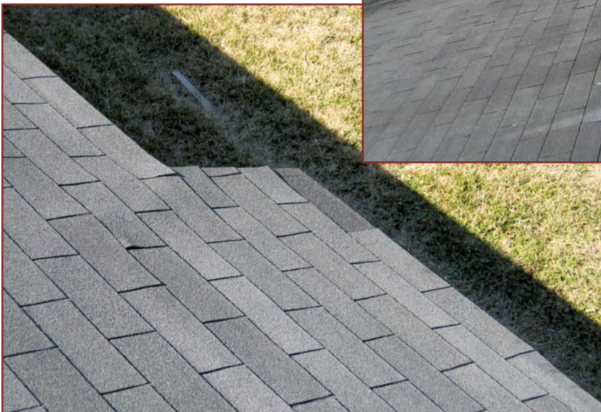
Above: Photo 9 – Less extensive wind loss of shingles occurred with the “moderately old” shingles, primarily near the roof perimeter, such as on Building 18.
