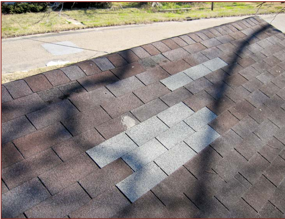
Photo 11 – Despite overexposure, repaired portions of “old” shingle roofs performed well during the hurricane, such as these repairs on Building 13.
