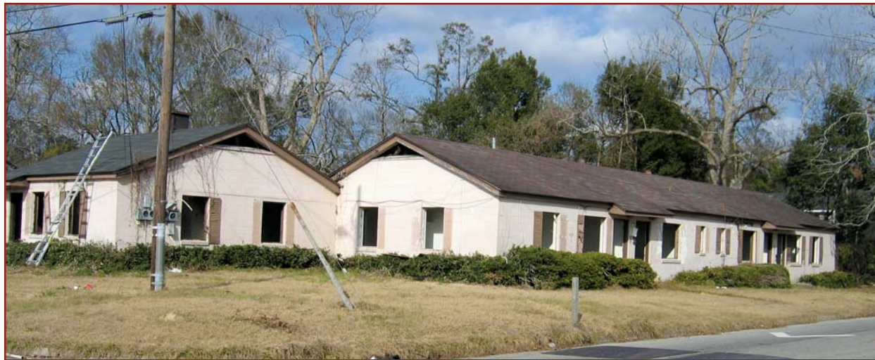
Photo 1 – Typical configuration and condition of building structure within the housing complex.
