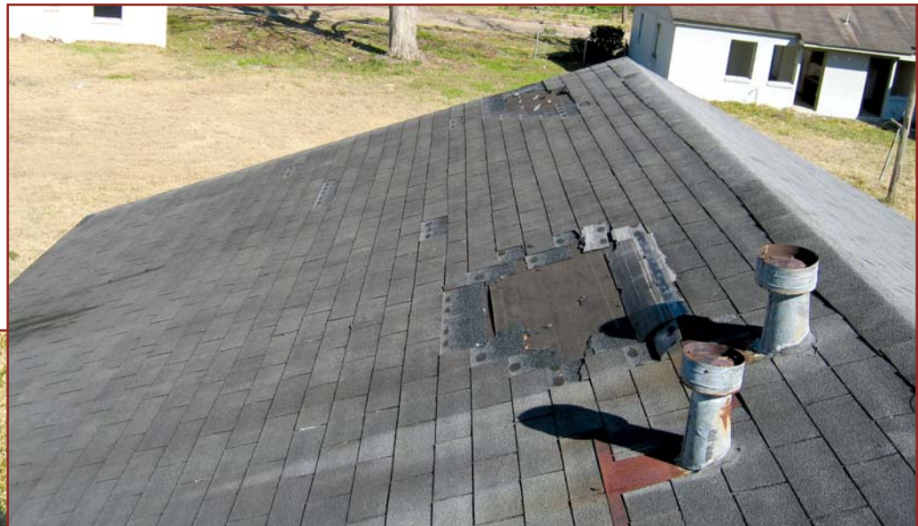
Above: Photo 9 – Less extensive wind loss of shingles occurred with the “moderately old” shingles, primarily near the roof perimeter, such as on Building 18.
