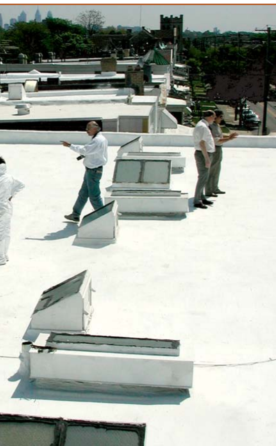
Photo 4: Overview of several residential roofs.
