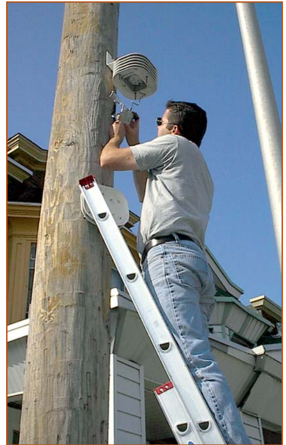
Photo 6: Installing data loggers for “cool block” comparison.
