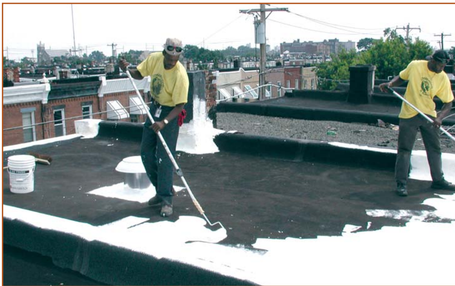
Above: Photo 1: Application of elastomeric acrylic roof coatings to residential roofs.
