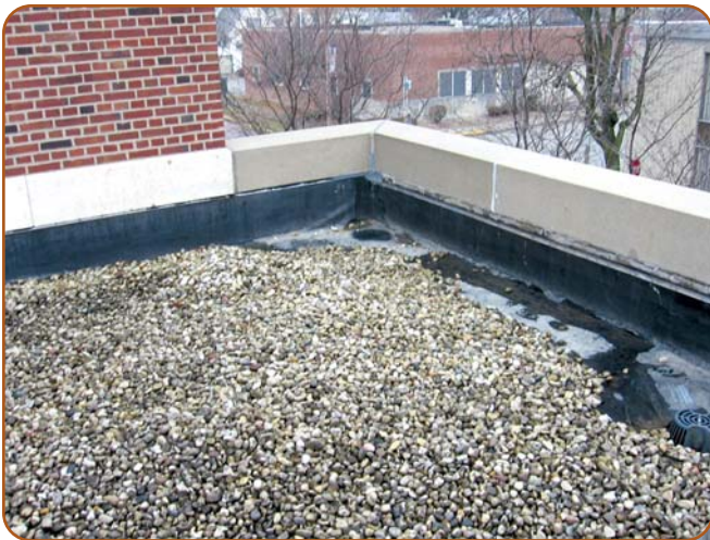
Above: Roof perimeter showing coping stone.
