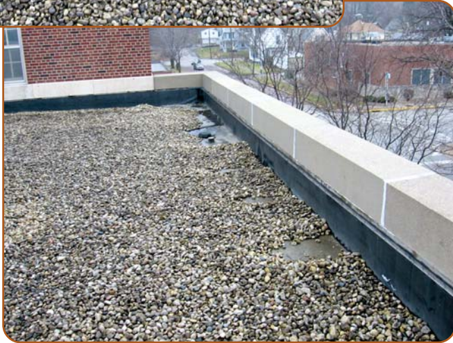
Right: Overview of roof edge.
