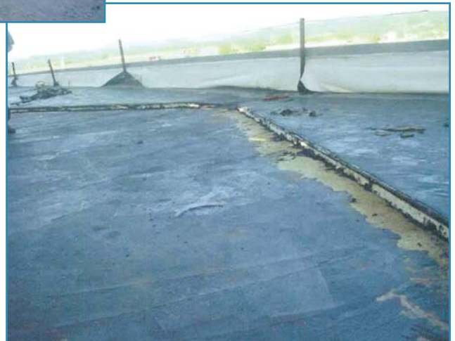
Figure 4 (above) and Figure 5 (right): Poor adhesion of primer over a wet concrete substrate. Long night seals can be sources of water under newly installed roof assemblies.
