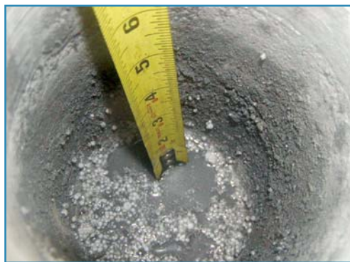
Figure 3: Core into a concrete slab to the steel pan below.
