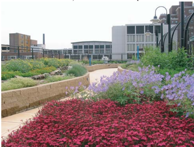
Schwab Rehabilitation Hospital - Chicago, IL (2005 Green Roof Awards of Excellence winner)
