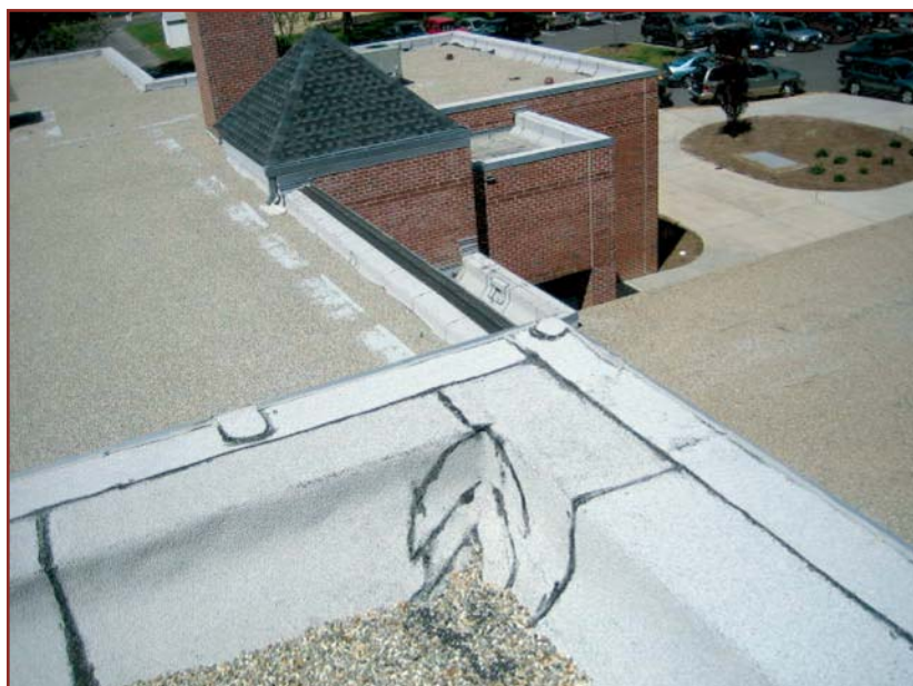
Figure 5. Flashing details are critical to the long-term performance of any roofing system.
