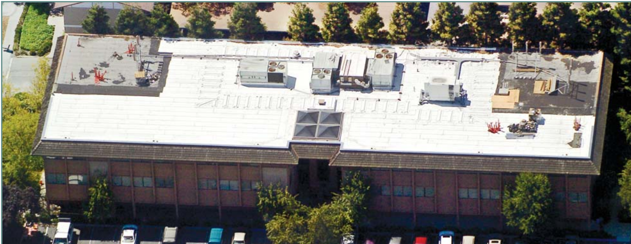
Factory-coated BUR cap sheet on Armado Plaza, Dublin, CA.
