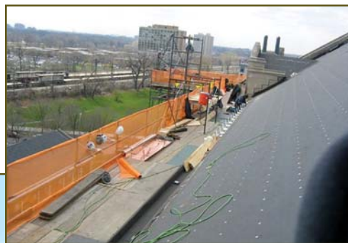
Right and Below: Scaffolding provides safety from falling debris to those below. Photo by Knickerbocker Roofing.
