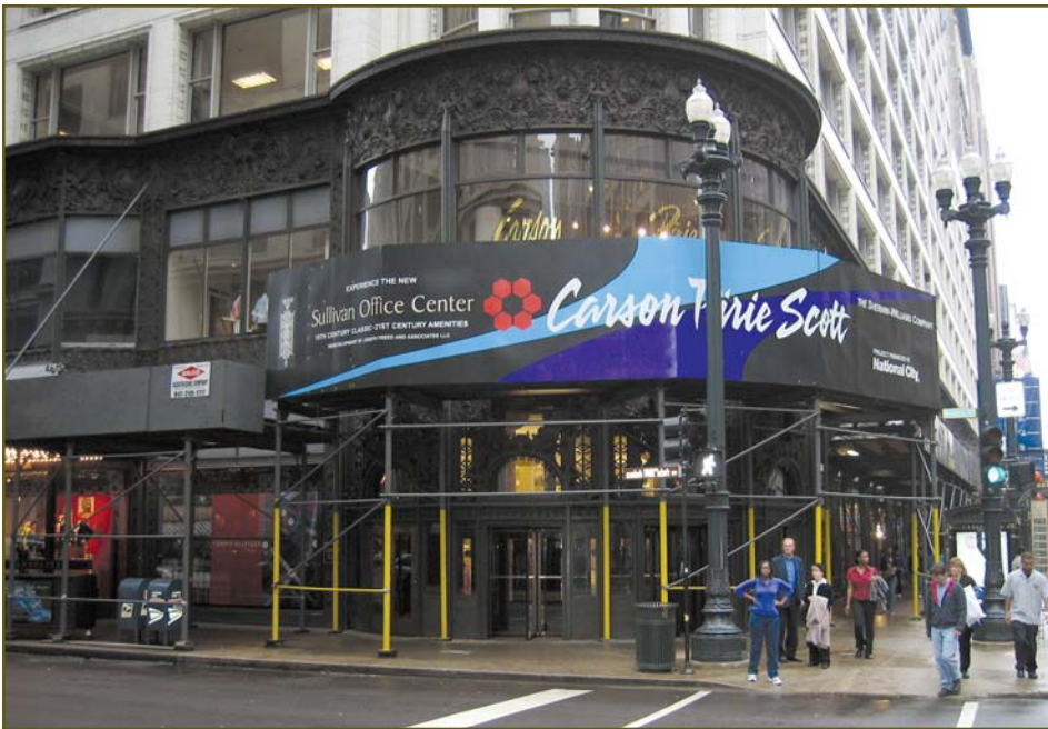
Scaffolding allows building operations to continue while work takes place above. Photo by Knickerbocker Roofing.
