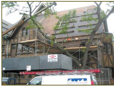
Scaffolding secures residence from damage.
