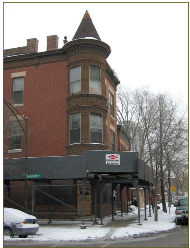
Scaffolding keeps retailers open.
