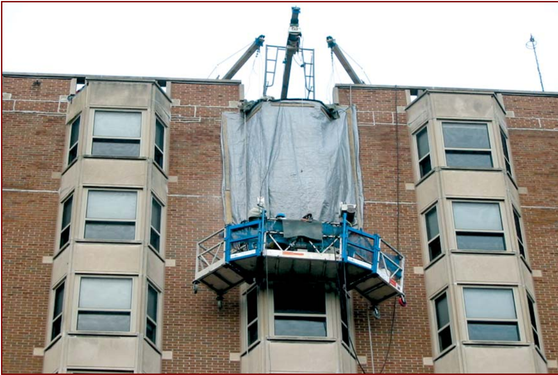
Figure 5 – Large-scale selective removals of cladding features.
