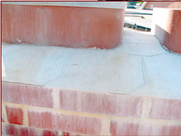
Left: Figure 11C – Latent defects in mortar-topping material contributory to the cause of the efflorescence and spalled brick (2004).
