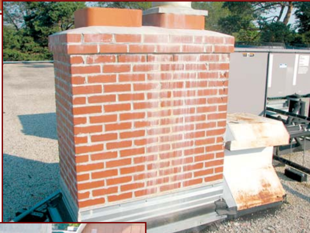
Left: Figure 11C – Latent defects in mortar-topping material contributory to the cause of the efflorescence and spalled brick (2004).
