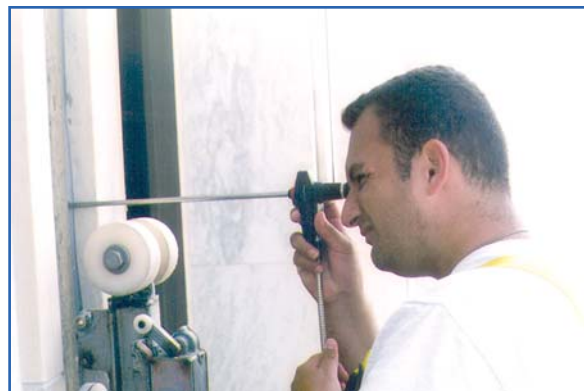
Figure 3 – A fiber optic borescope is used to view inside a building façade. Borescopes require small holes in building façades in order to peek inside the wall system.
