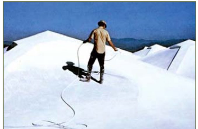
A new generation of elastomeric, acrylic coatings provide reflection and UV protection to single-ply, bituminous, MB, SPF, and metal roof systems. In some re-cover applications, just acrylic coating and reinforcing fabric constitute the “no-ply” roof system.
