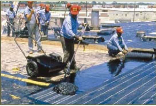
The traditional BUR uses three to five plies of reinforcing, with each ply laid in hot asphalt.
