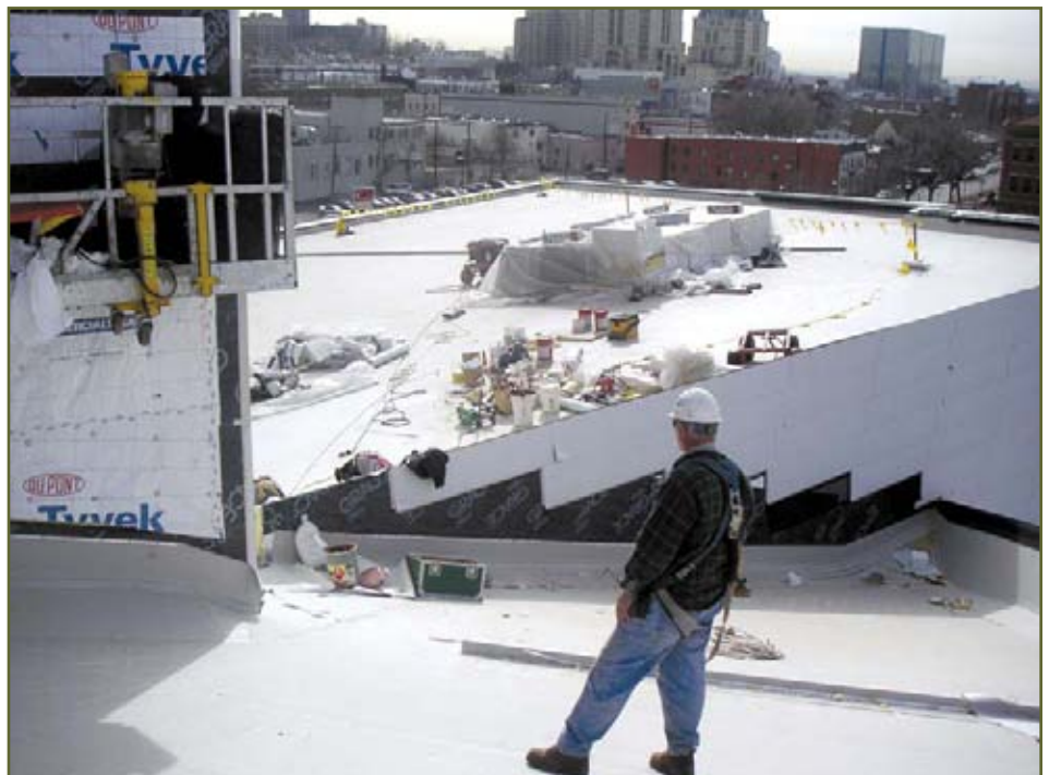
While called a single-ply system, all thermoplastic systems use internal reinforcement with polymer layers on both sides of the fabric.
