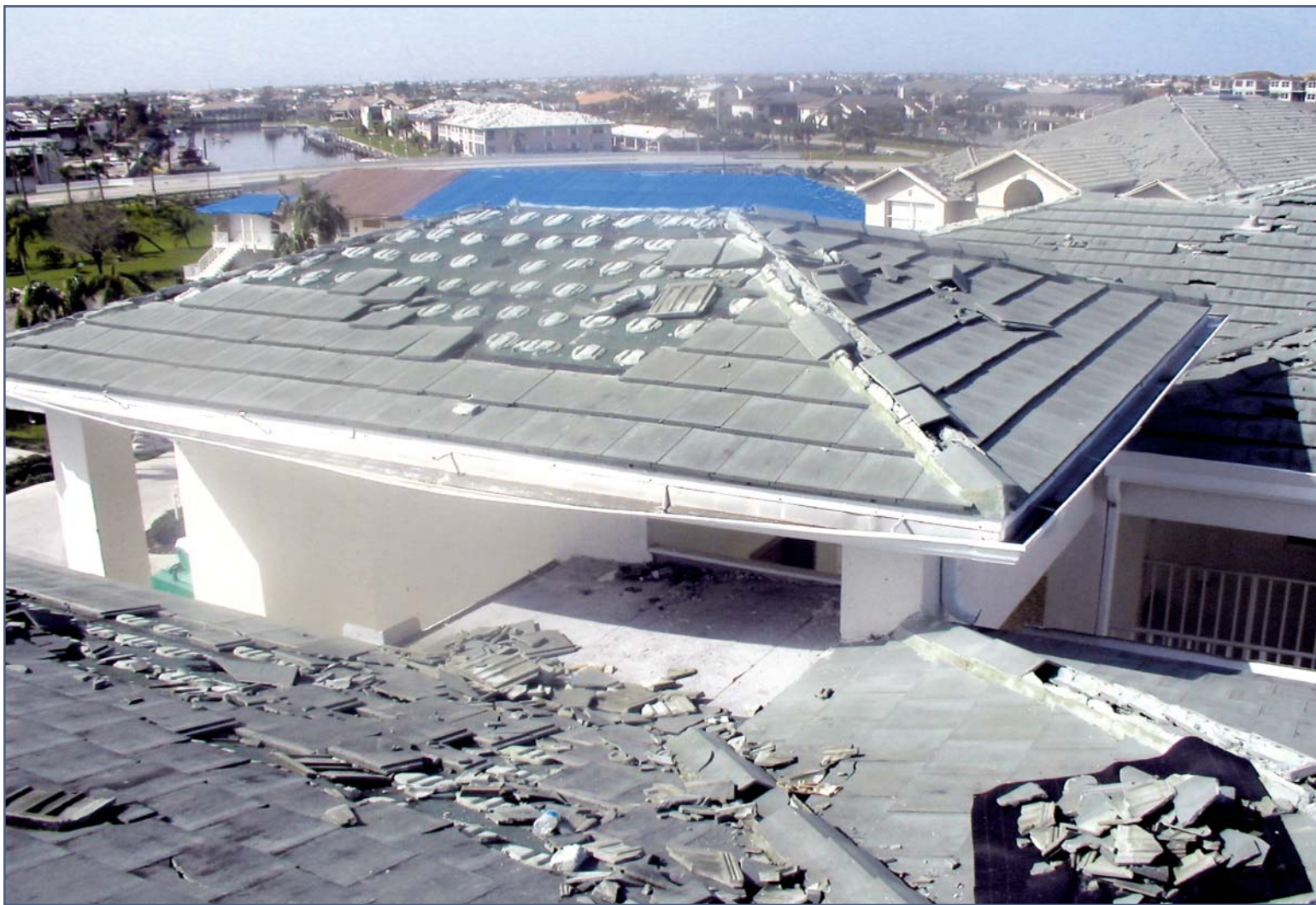
Photo 5 – Example of a ridge tile failure in a concrete tile roof system. Photo courtesy of Warren French.
