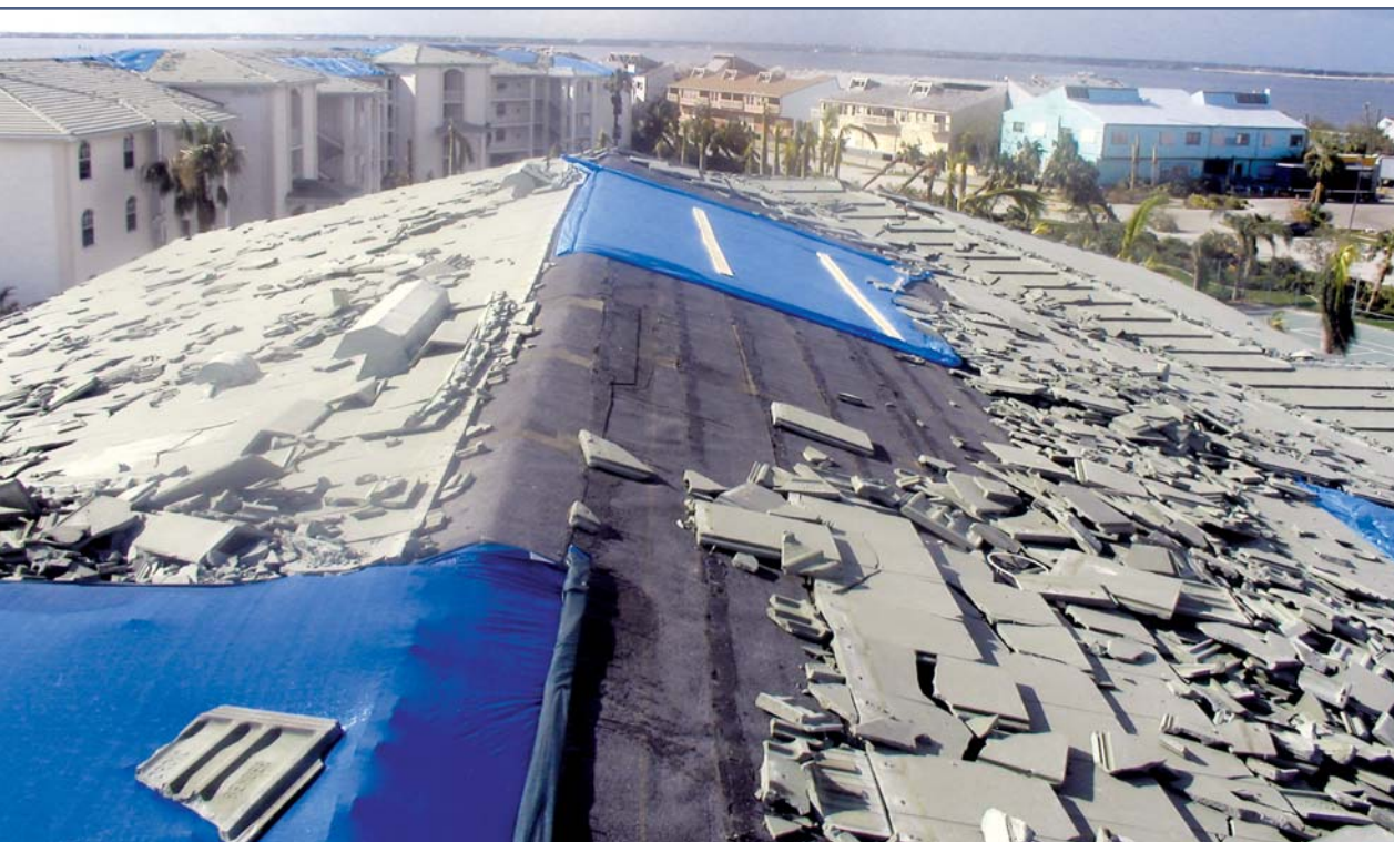
Photo 6 – Upper concrete tile roof exhibiting partial failure of the “foam-set” system, possibly due to an improper foam mix. Lower roof exhibiting damage from flying debris. Photo courtesy of Warren French.
