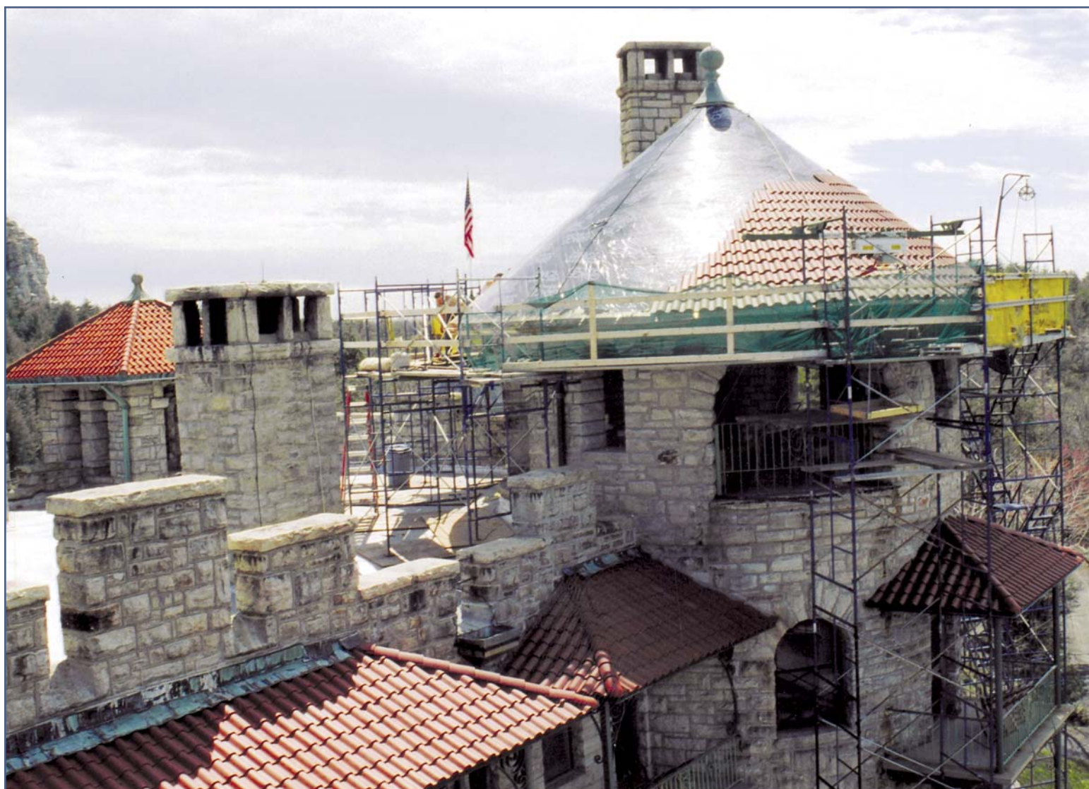
Photo 3 – Process of replacing original Ludowici Celadon clay Spanish tile (initially installed at the turn of the 20th century) with new tile by the same manufacturer on an historic hotel in upstate New York (the original tile came from Celadon's plant in Alfred, NY). Photo by Robert L. Fulmer.
