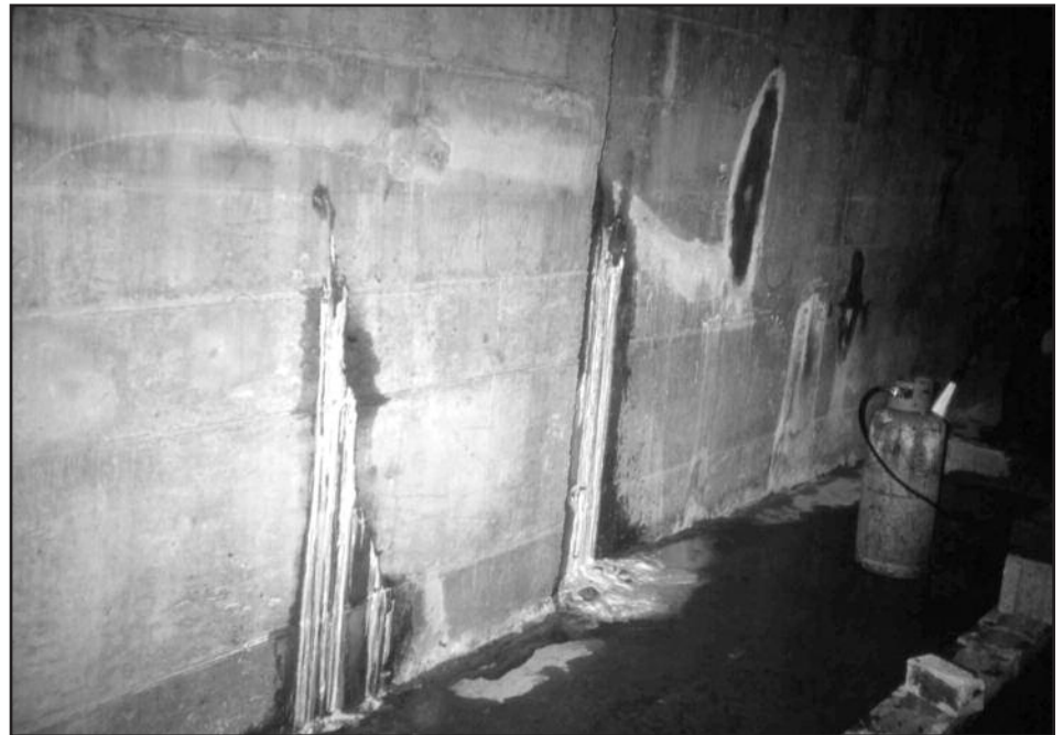
Photo 1 - Below-grade leak.
