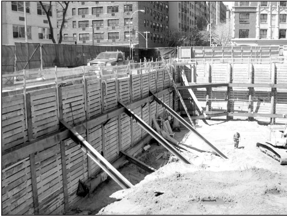
Photo 3 – Earth retention system.
