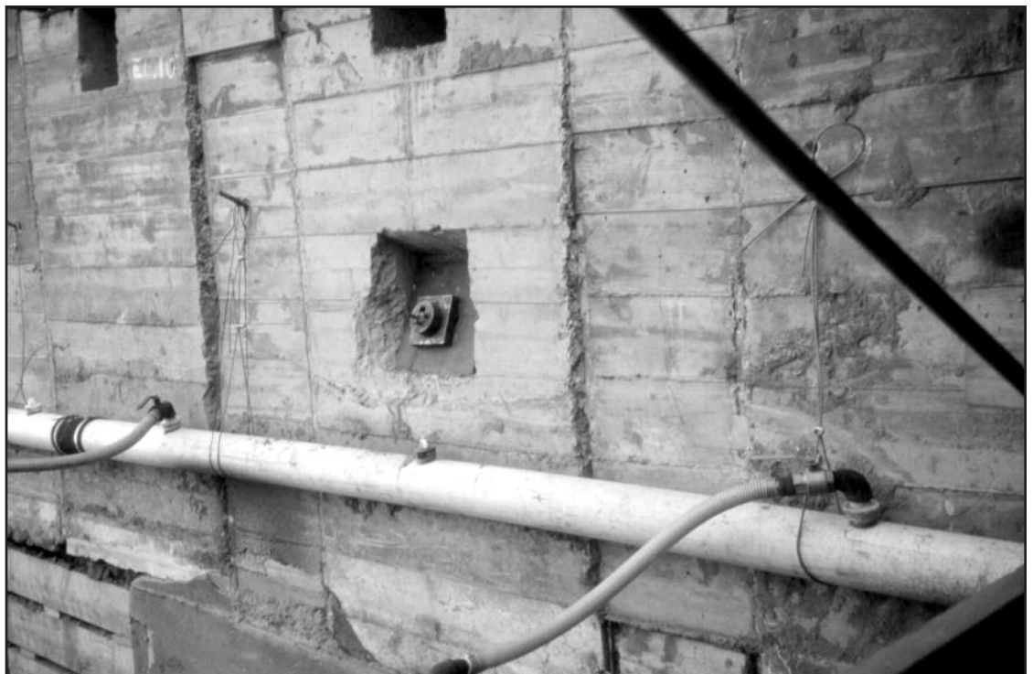
Photo 4 – Site dewatering system.
