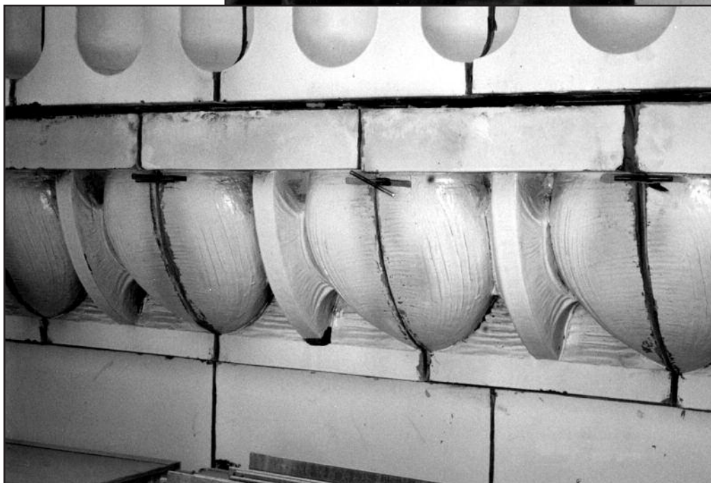
Figure 7 – Anchor rods slotted into terra cotta units.
