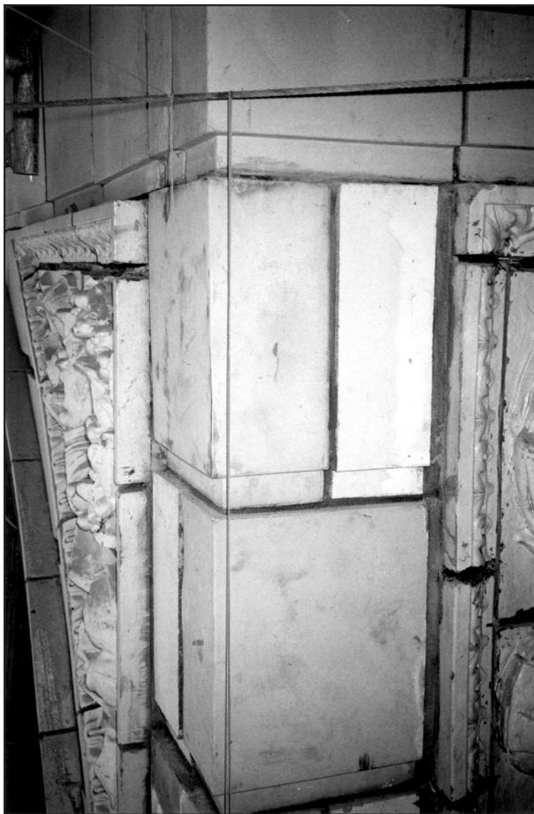
Figure 5 – Concrete replacement units around original terra cotta unit.
