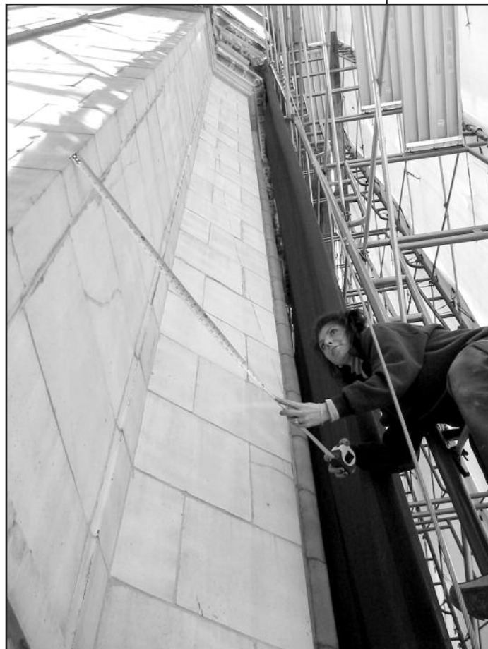
Above: Figure 4 - Roof measurements obtained with use of a pole and plumb-bob.
