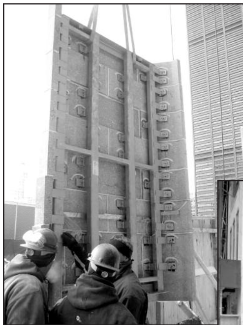
Figures 22A and 22B – New steel tube panels with stone facing installation.
