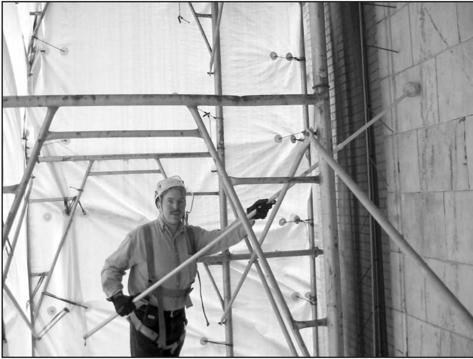
Figure 8 – North elevation – sounding of terra cotta with “sounding ball.”
