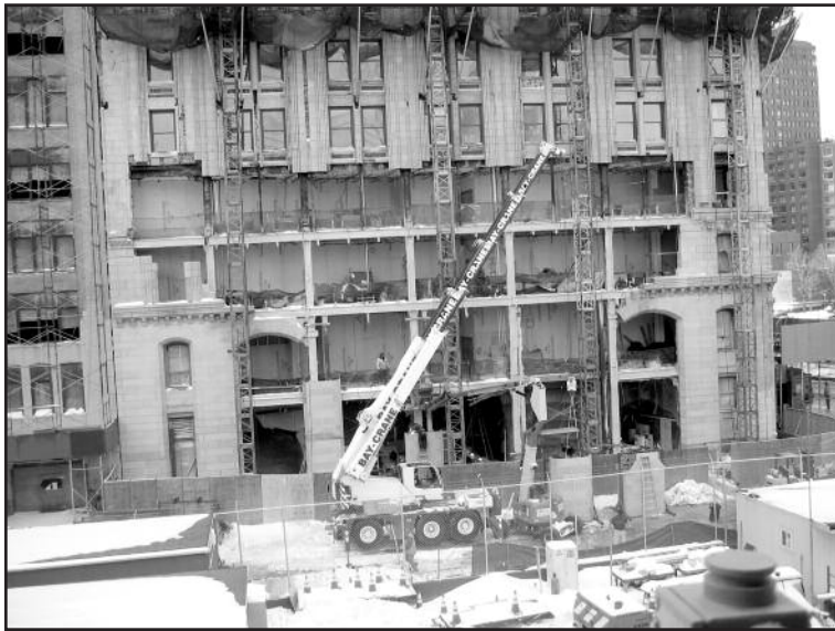
Figure 19 - North base - most of the north façade granite was completely removed.
