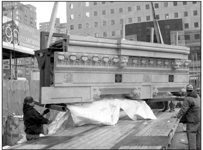
Figure 23 – Granite panel hoisted from flatbed truck.
