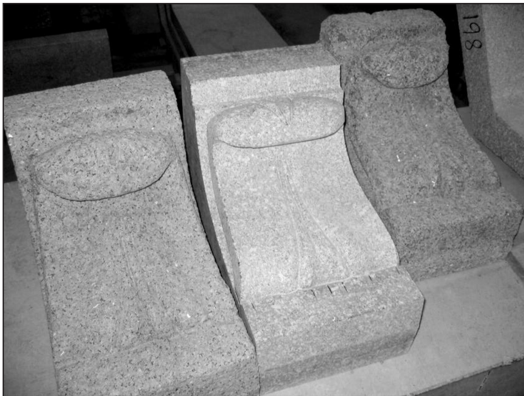
Figure 21 – Existing and new granite bracket during fabrication.
