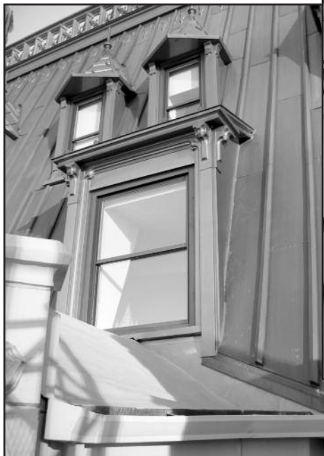
Figures 15A and 15 B – Completed mansard roof with new fiberglass balustrade and icicles.
