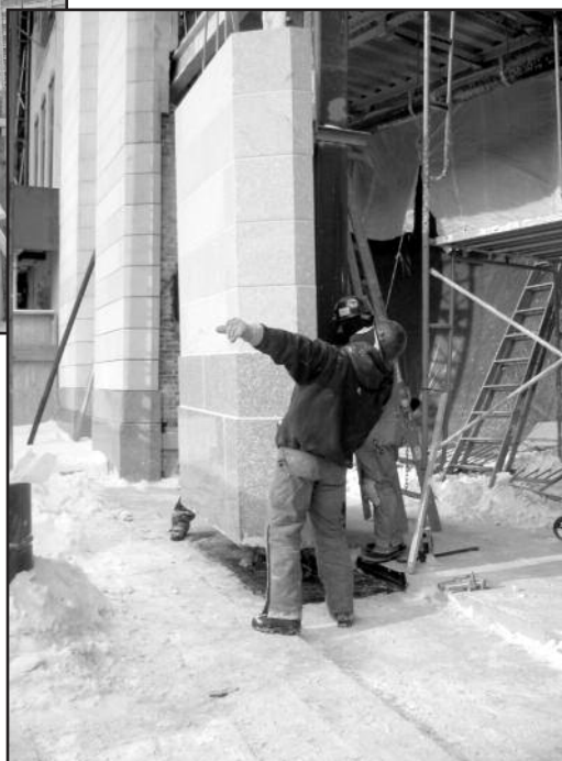
Figures 22A and 22B – New steel tube panels with stone facing installation.
