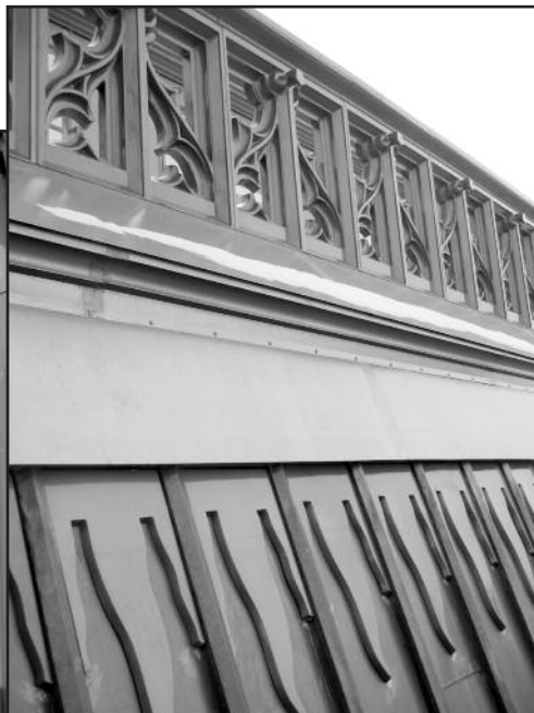
Figures 15A and 15 B – Completed mansard roof with new fiberglass balustrade and icicles.
