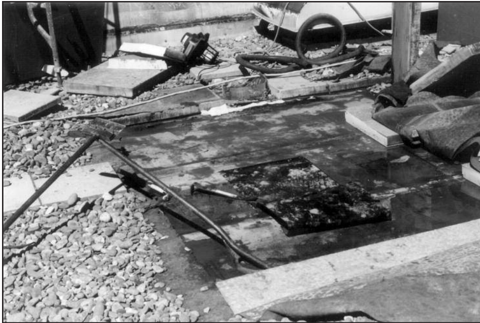
Figure 6 – Test opening in existing IRMA roof system.
