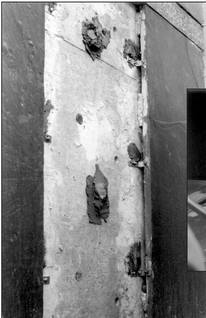
Figure 25 - Reinstallation of slate wall panels.
