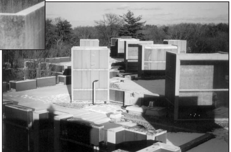
Figure 5 – View of roof prior to rehabilitation.
