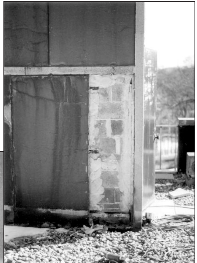
Figure 8 – Test opening at stair tower wall.
