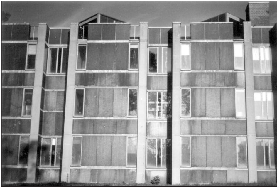
Figure 27 – East elevation prior to rehabilitation.
