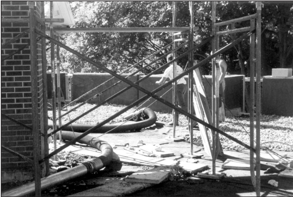
Figure 22 – Vacuum removal of ballast in progress.
