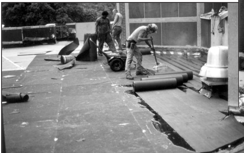
Figure 7 – Installation of new roofing system.
