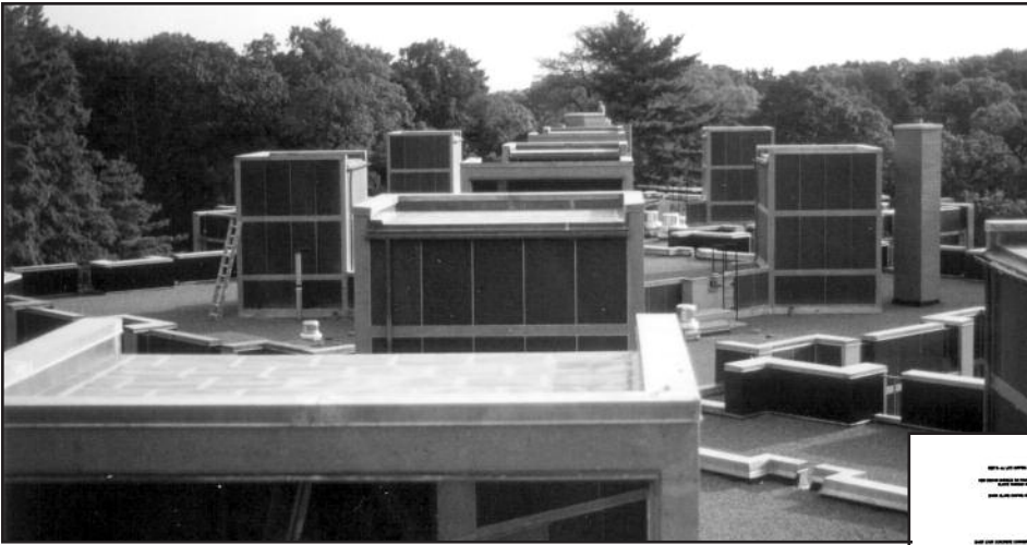
Figure 15 – New clerestory roofing.
