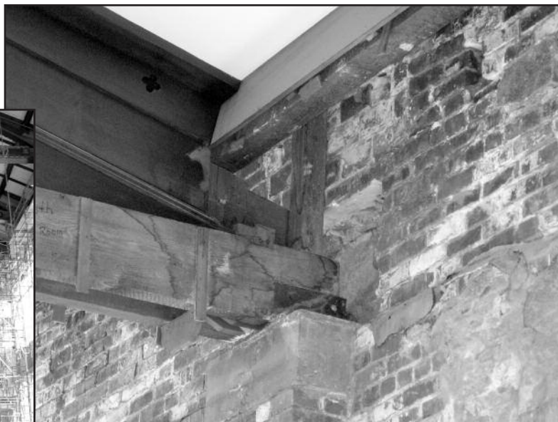
Figure 11 – Removal of masonry from truss ends to isolate wood from masonry.
