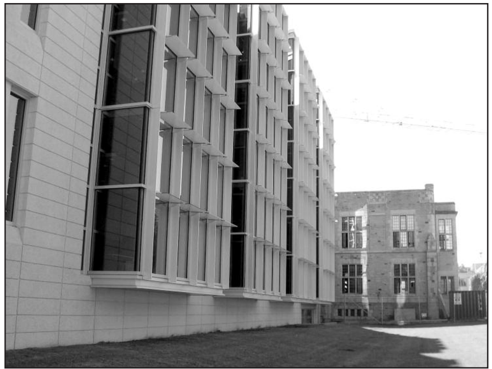
Figure 6 – View of new wing with heritage core beyond.
