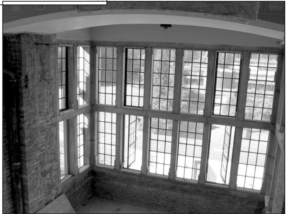
Figure 4 – Original steel-framed windows in set-in granite mullions.
