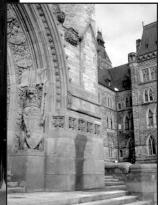
Below: Figure 4 – Water-shedding details deflect water off the upper surface of the masonry. Unfortunately, the water is deflected onto lower surfaces.
