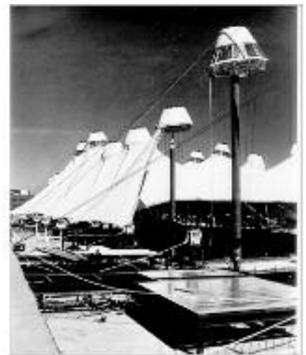
Partially-completed tensile membrane roof.
