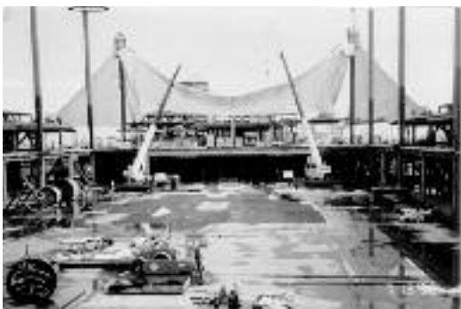
Fabric was lifted into place with a drum hoist (in foreground) secured on the terminal's Main Level 5. Two hydraulic cranes were also used to assist with the lifts.
