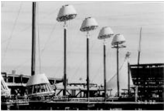
Steel masts were guyed with external temporary cables, and truss rings were assembled around mast bases and winched up into position.
