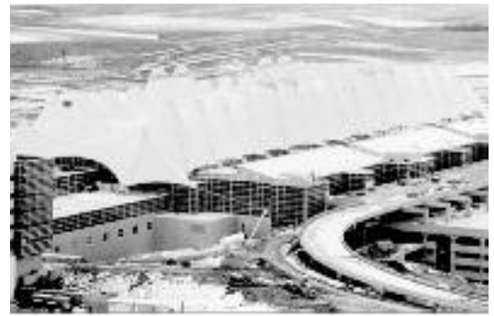
Aerial view of the Jeppesen Terminal's tensile membrane roof.
