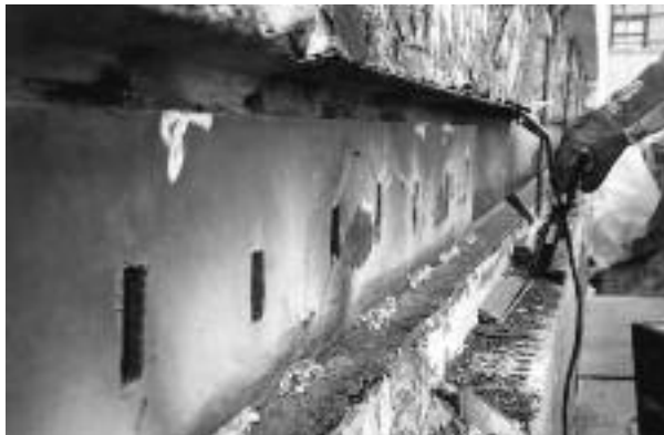
Figure 11 – New steel plate being welded to existing beam.
