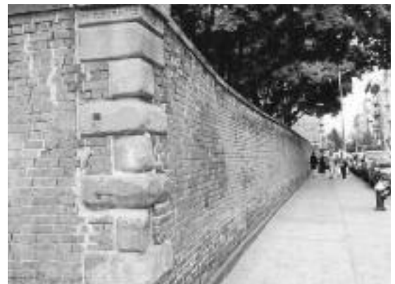
Figure 4 – Bowing due to restrained thermal movement.
