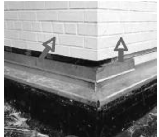
Figure 10 – New through-wall flashing at setback wall. Note header brick course (arrows).
