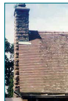
Figure 2: This roof, on a golf course clubhouse in South Africa, shows that Gloeocapsa Magma is as much at home in Africa as North America. Also note the effect of the copper flashing around the chimney. (Courtesy, Michael Rosenthal, Durban, South Africa.)
