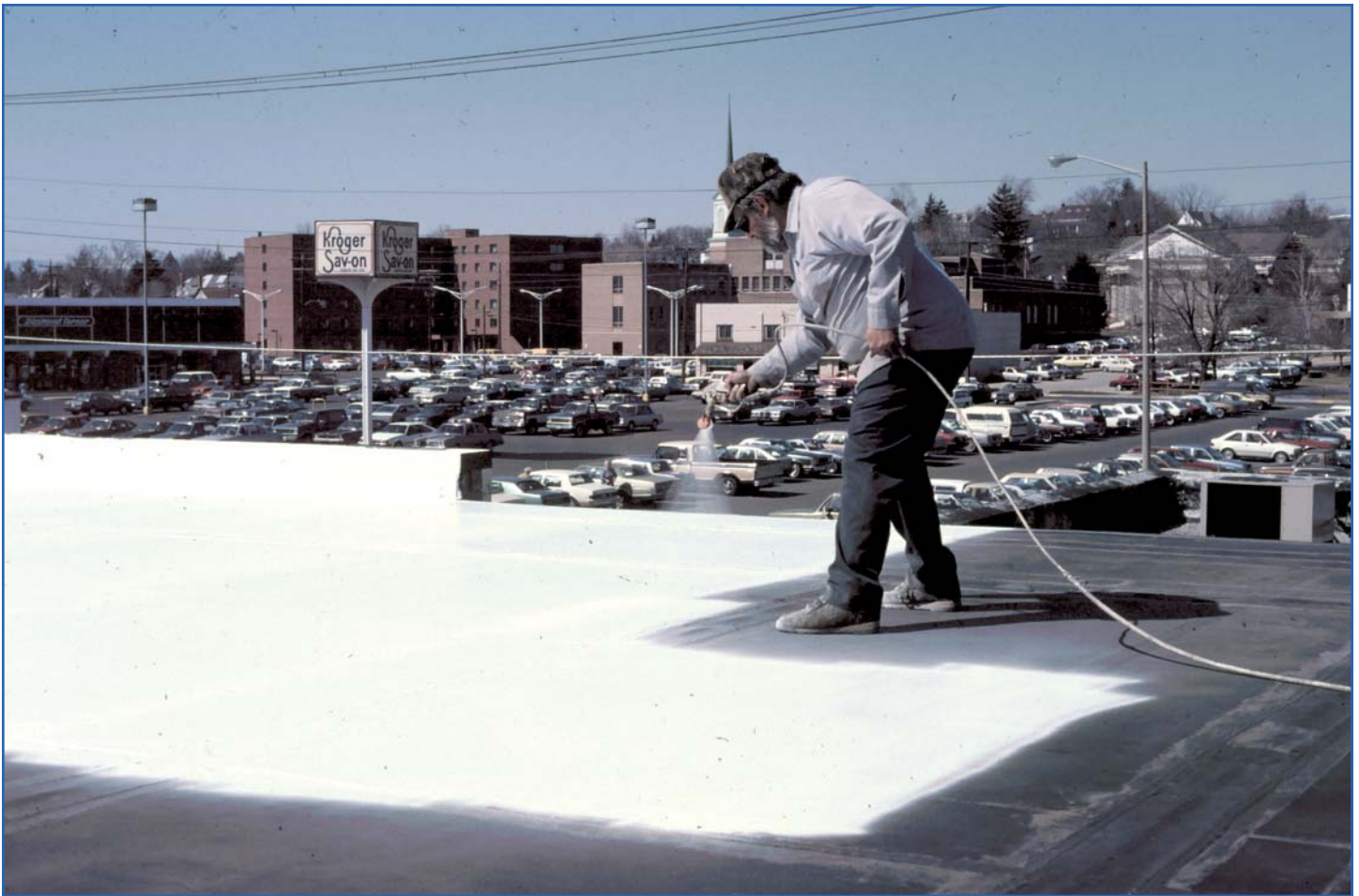
Roof coating being applied.
