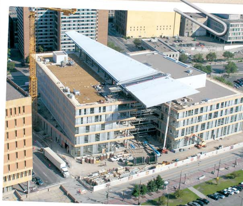
Project in progress, before green roof installation.
