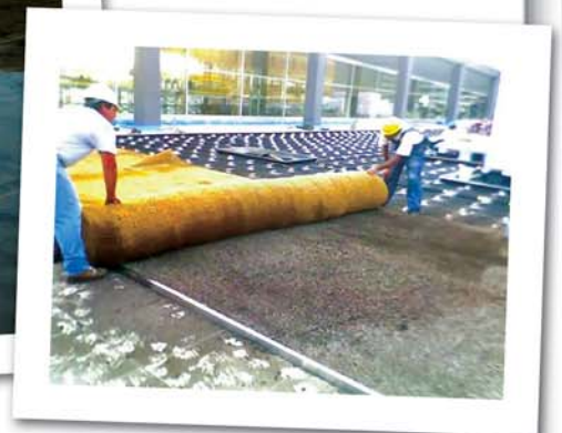
Installation of a coconut windscreen over the growing medium.
