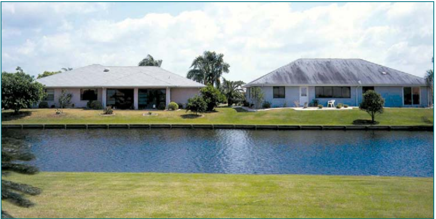
Figure 3: The Scotchgard™ Algae Resistant (AR) Roofing System from 3M for asphalt shingles, shown on the home on the left, combines a defined percentage of 3M copper granules with 3M standard colored granules to help provide effective protection against algae growth. Algae have stained the untreated shingles of the house on the right. (Courtesy of 3M.)
