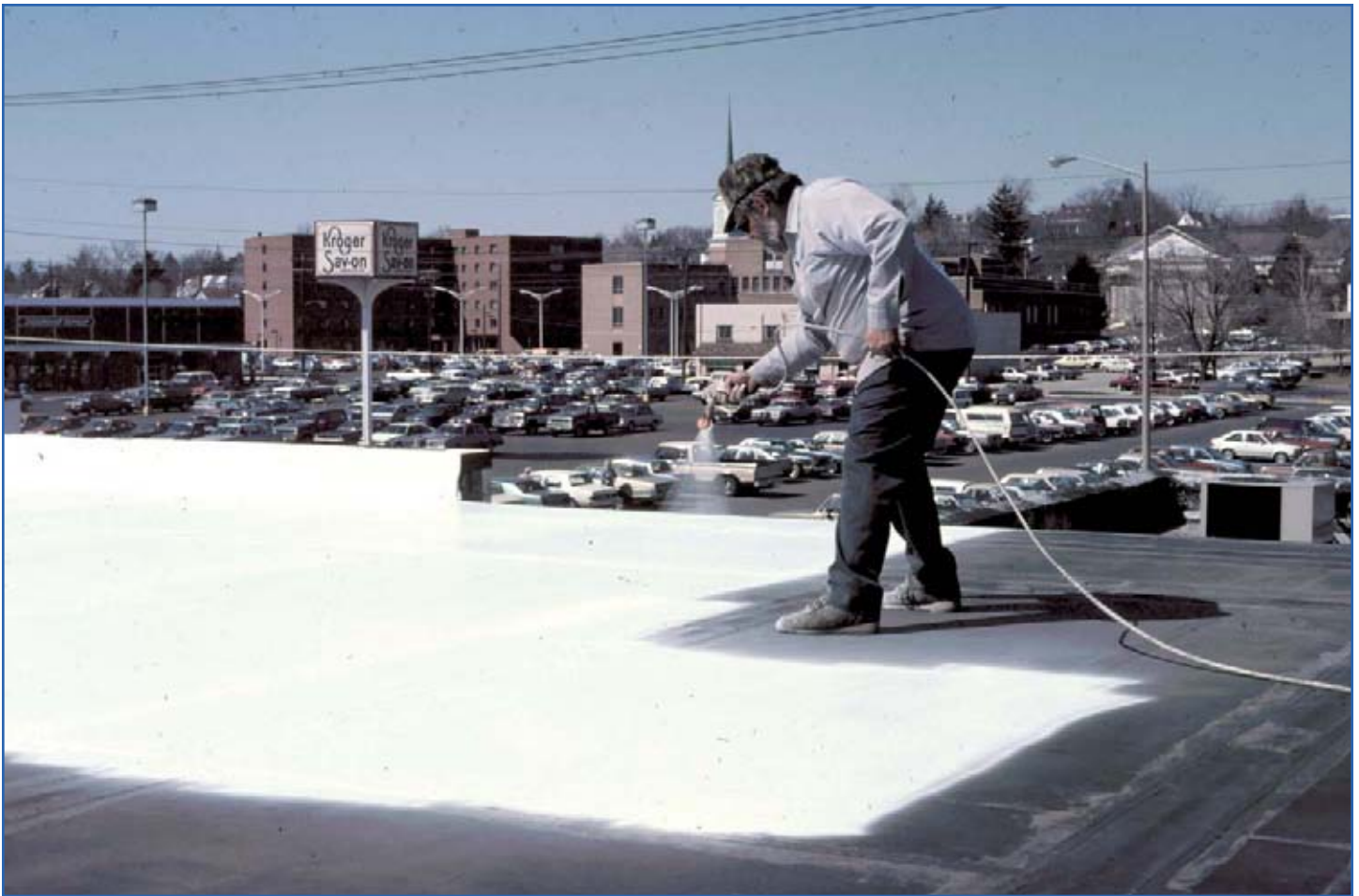
Roof coating being applied.
