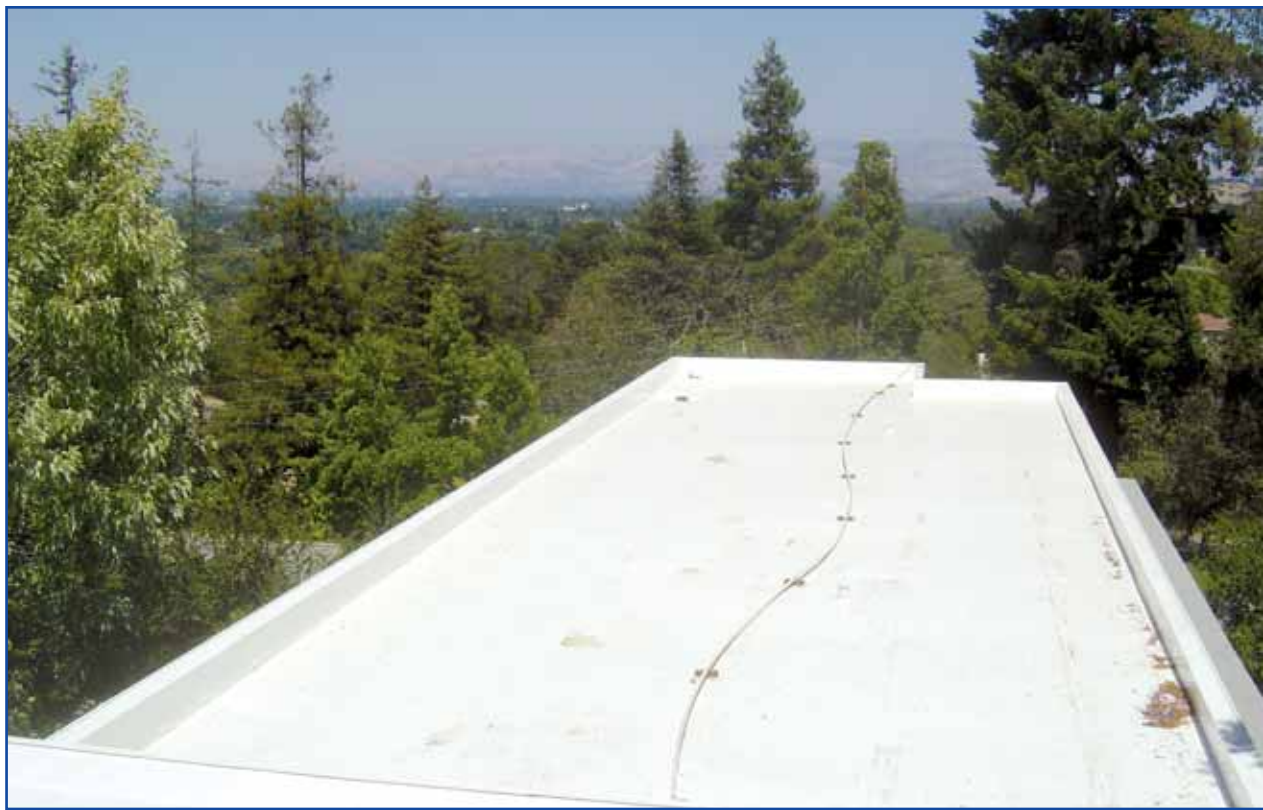
Photo 1 – Typical Title 24-compliant single-ply roof.
