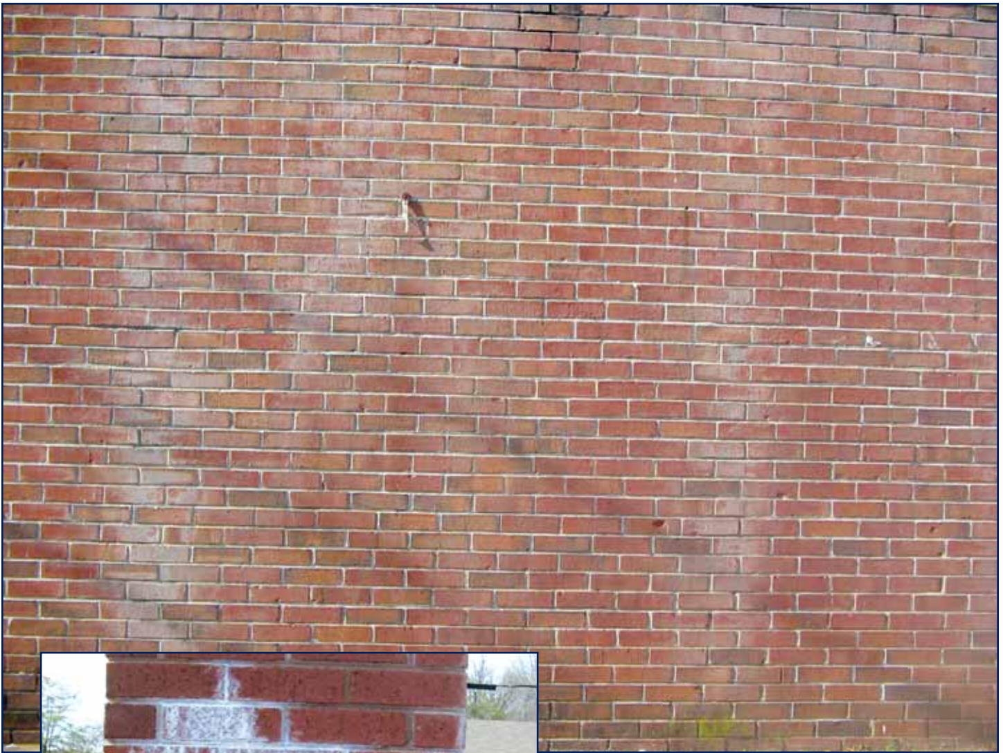
Figure 4A – Mild efflorescence on brick.
