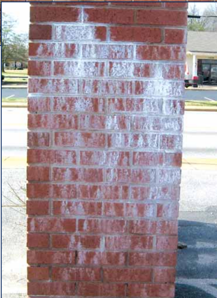
Figure 4A – Mild efflorescence on brick.
