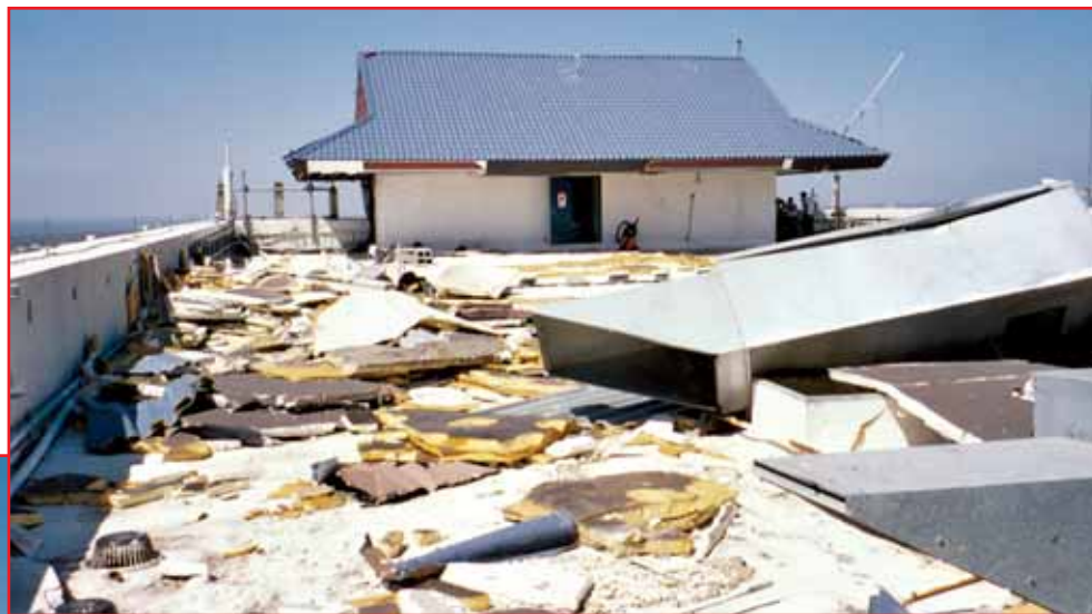
Photos 1 and 2 – Impact of reduced fastening patterns.
