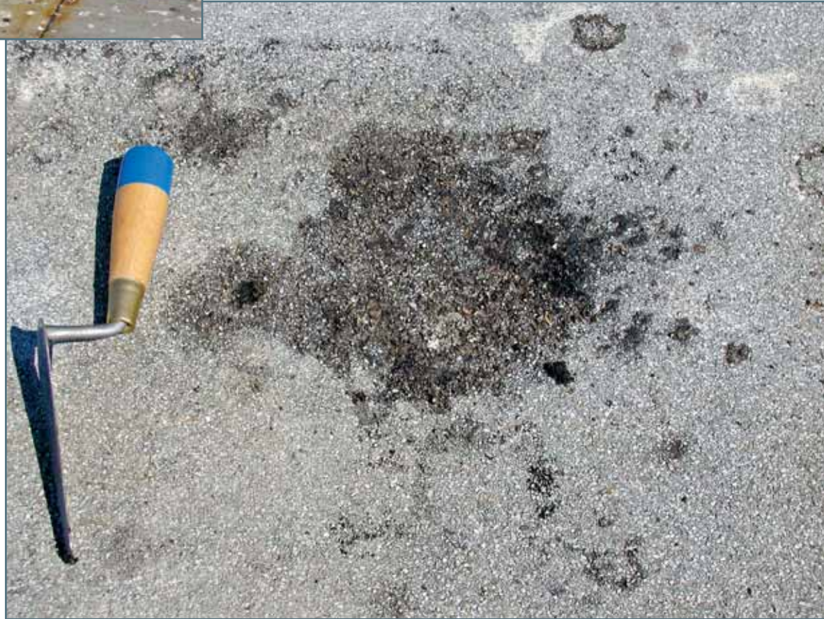
Photo 3 – This picture demonstrates damage to the membrane that almost reaches the reinforcing mat. Granular degradation is devastating; the asphalt blend is softened and contaminated.
