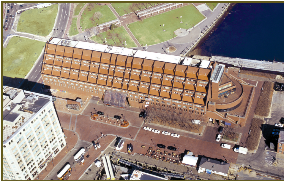
Figure 2 – Marriott Long Wharf with new roof.
