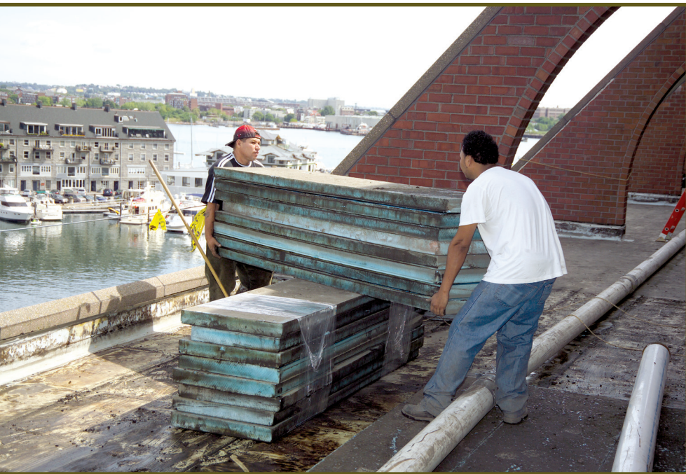
Figure 5 – The extruded polystyrene was re-used at other locations.
