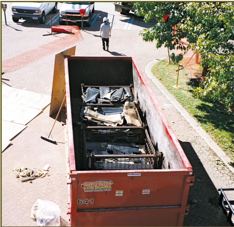
Figure 9 – Old membrane packaged in dumpster for shipment.
