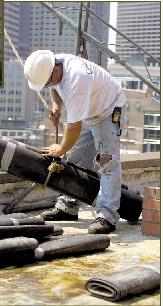
Figure 6 – Preparing the membrane for shipping.
