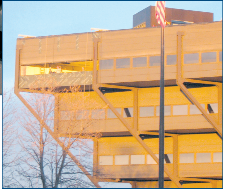
Photo 3 – Photograph of ribbon/strip windows; installation in progress.
