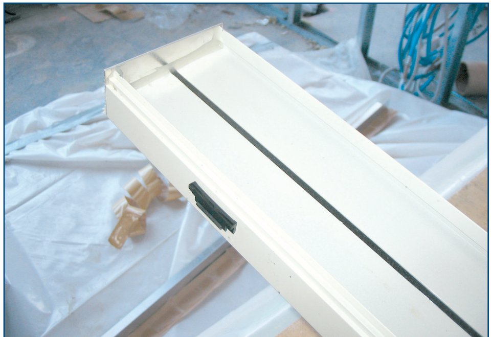
Photo 1 – Sample sub-sill with sealed end dam installed. Also note the black weep cover (which covers a slotted weep hole) and the slope to the exterior.
