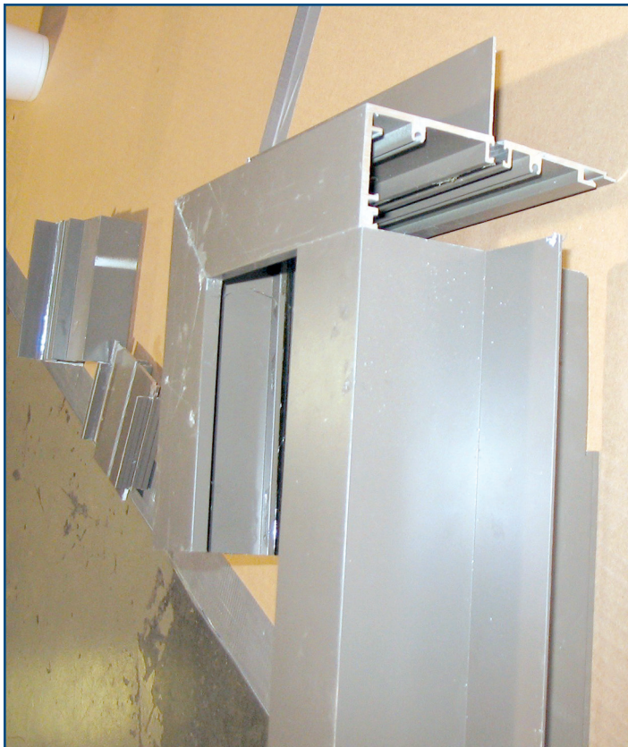
Photo 4 – Sample receptor frame intersection; note the open corner.
