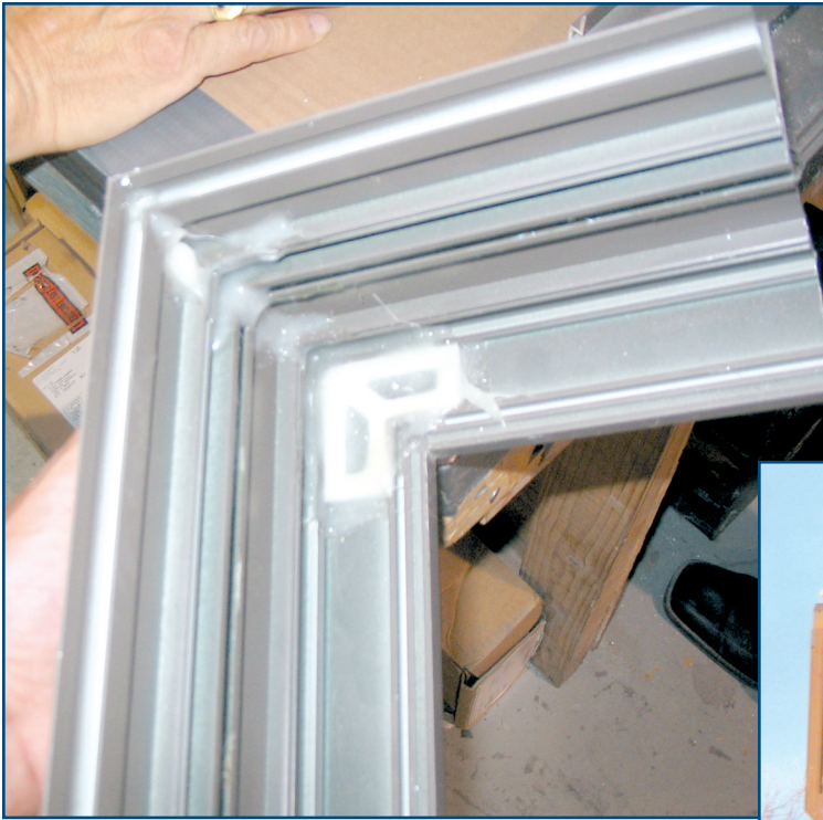
Photo 2 – Sample mitered receptor frame corner intersection; corner is keyed, fastened through screw bosses, and back-sealed.
