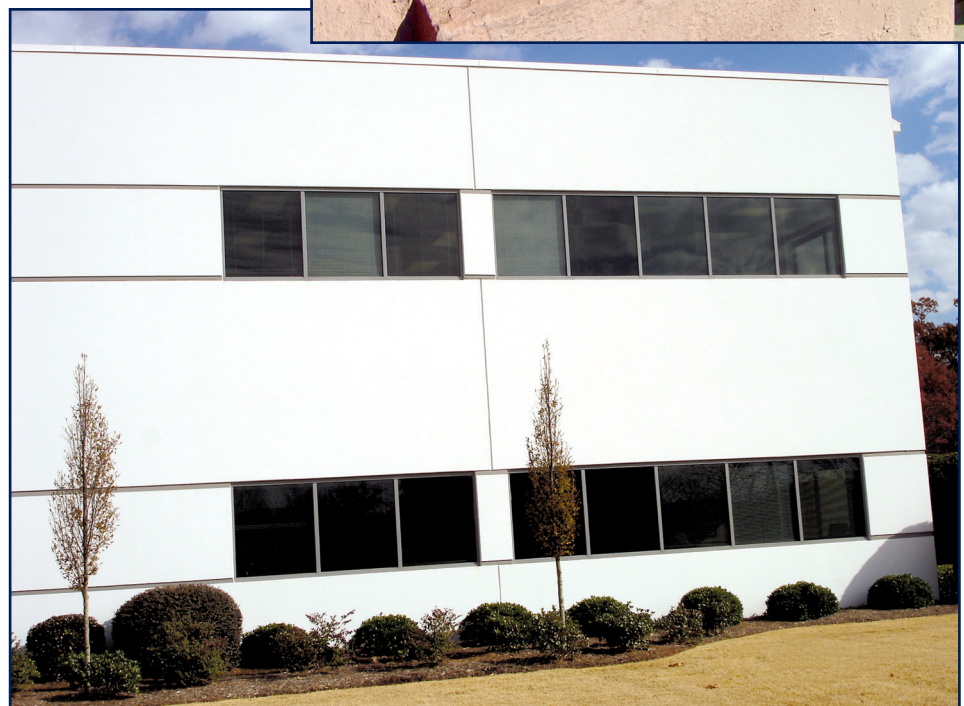
Figure 3-9 – Precast concrete coated with field-applied, acrylic-modified epoxy. Notice that the color is still vibrant after approximately nine years of weathering.
