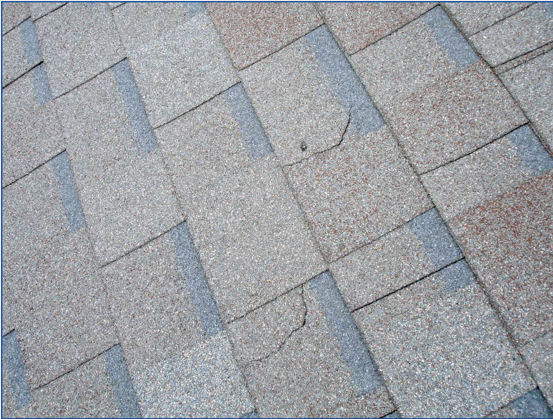
Photo 2 – Shingle splitting.
