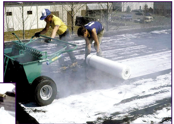
Figure 6: One layer of polyester mat laid in hot asphalt is a non-conventional single-ply roof membrane.
