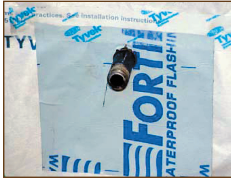
Figure 3: Penetration integrated into drainage plane.
