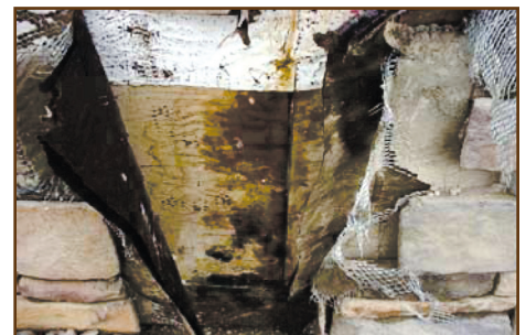
Figure 2: The consequences of reverse lapping.
