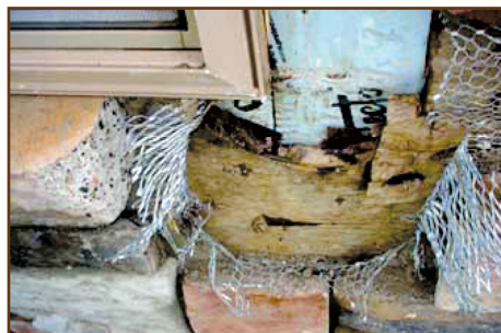
Figure 2: The consequences of reverse lapping.
