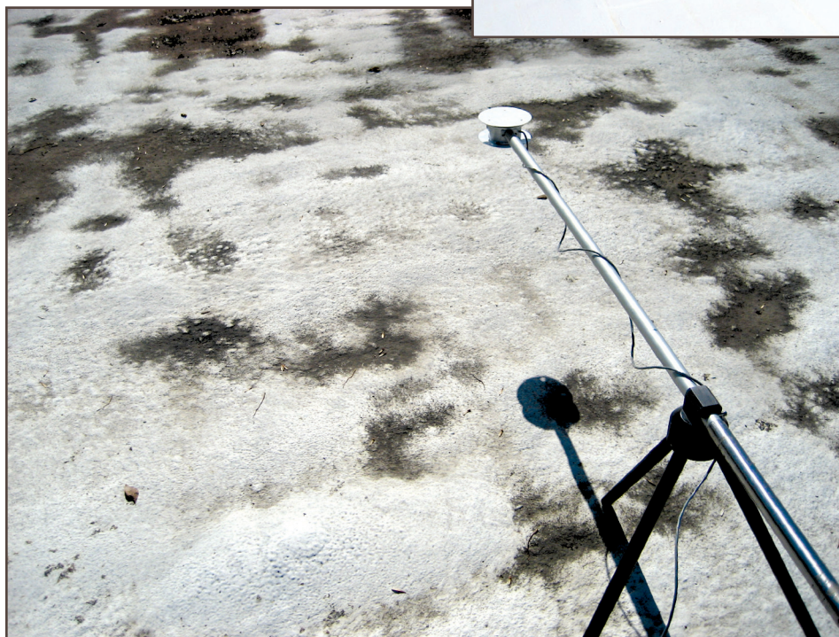
Photo 4 – SPF in Iowa, 3 years old, urethane/acrylic coating.
