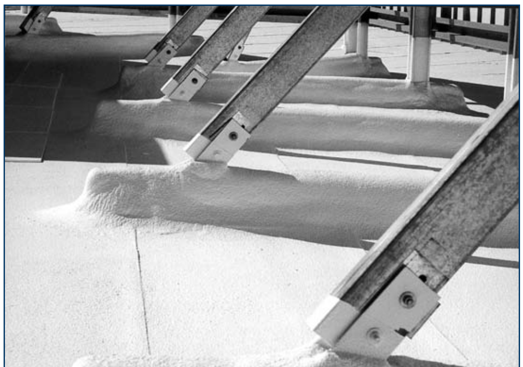
SPF roofing and restoration coating over BUR capsheet.
