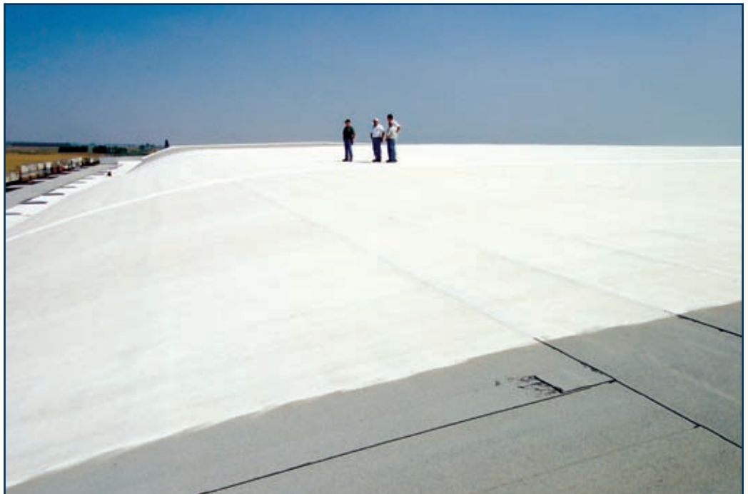
Modified-bitumen roof in the process of being coated.
