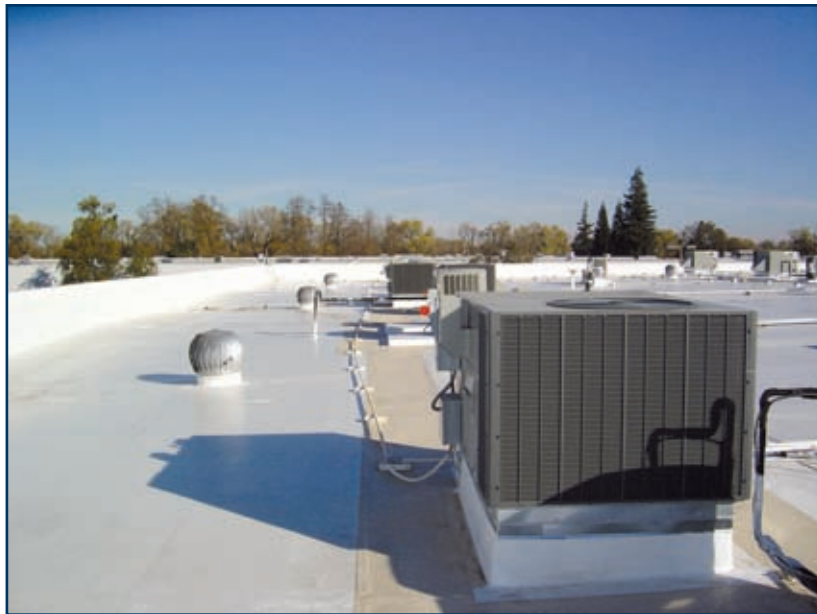
PVC coated roof.
