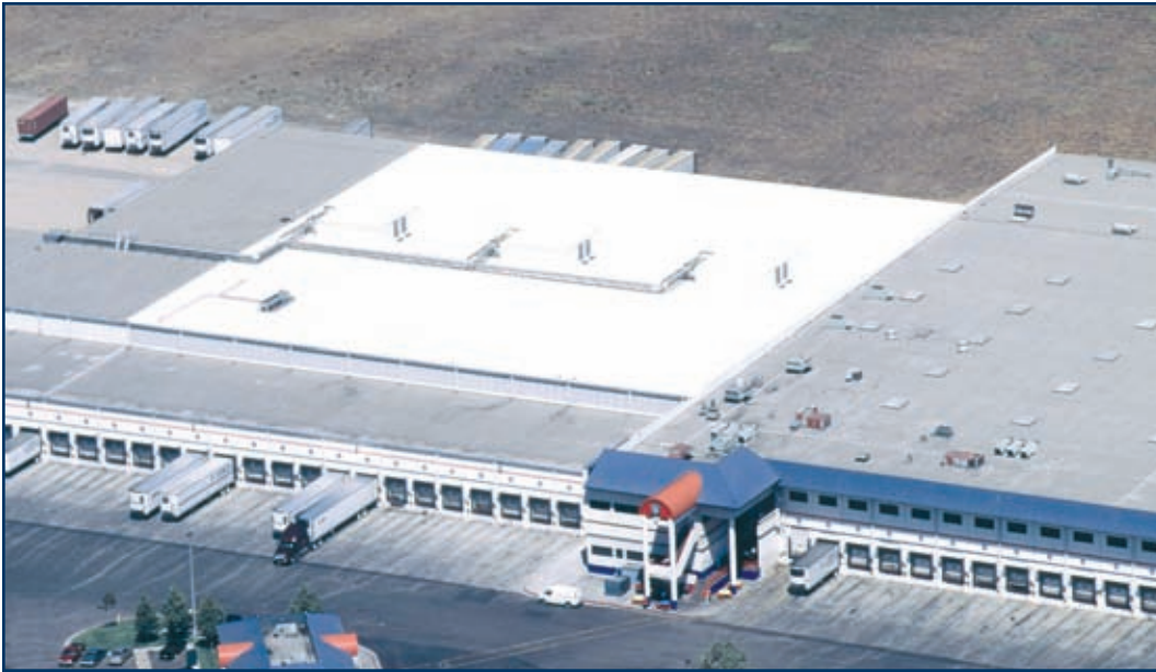
Reinforced coating system over BUR capsheet.
