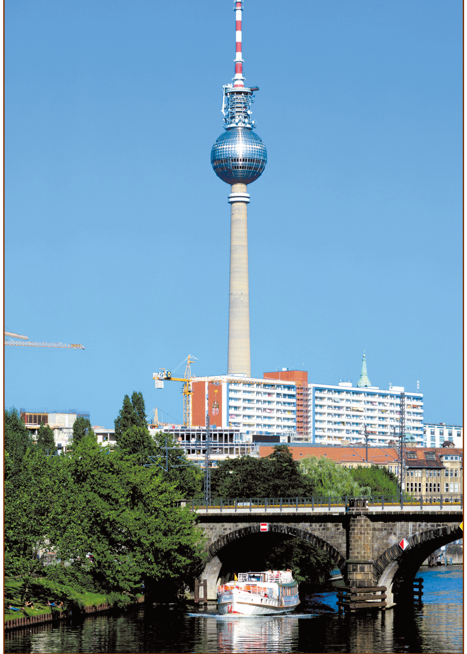
Alexanderplatz, the Berlin television tower built in 1969, presented waterproofing challenges. A strong bond was necessary between old concrete and repair mortar.
