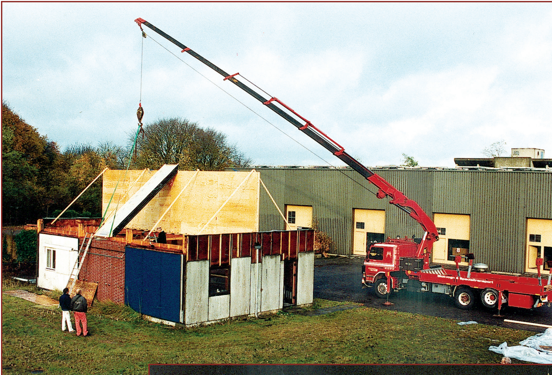
Figure 2 – Mounting of roof elements on the test house.
