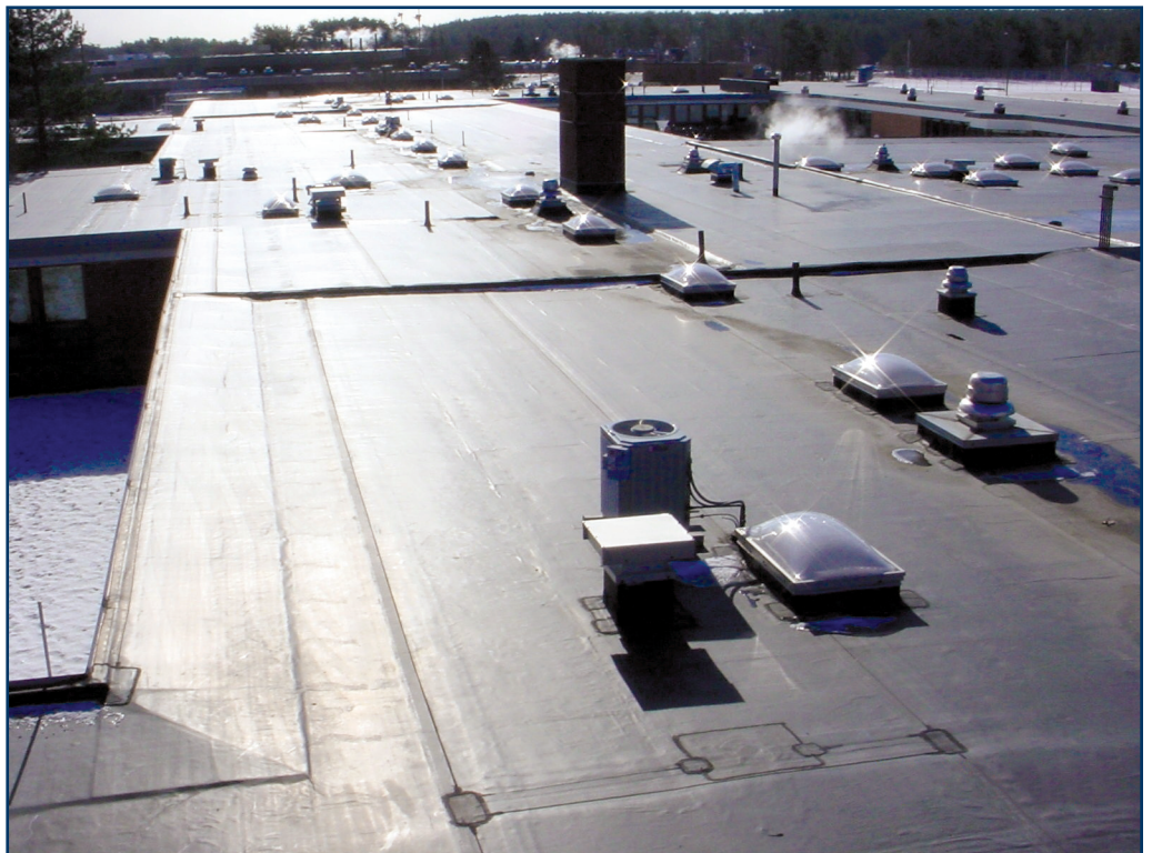
Finished view of Martinson Elementary School in Marshfield, Massachusetts. FleeceBACK applied directly over EPDM using FAST Adhesive made this roof as good as new.
