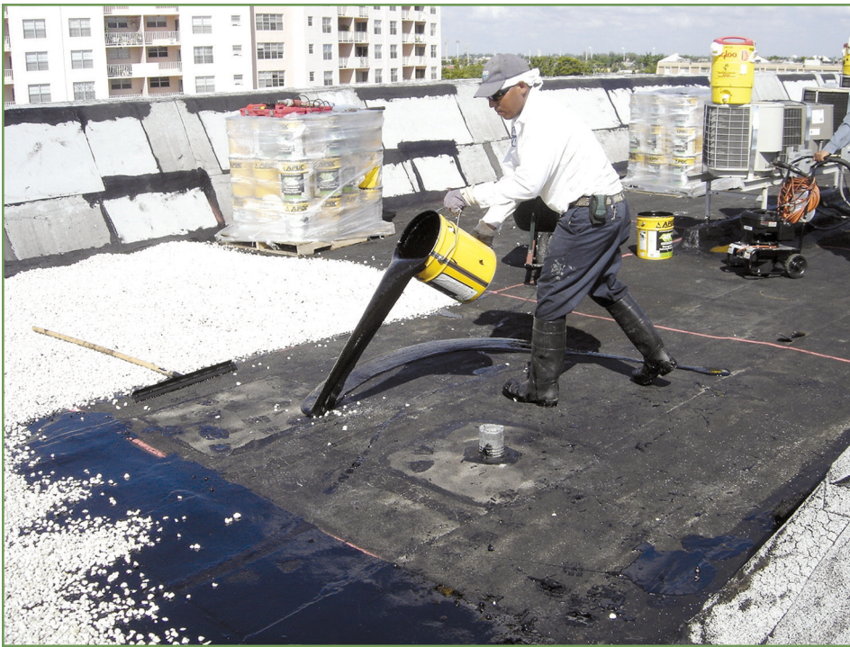
Application of a highly modified bituminous roof coating.
