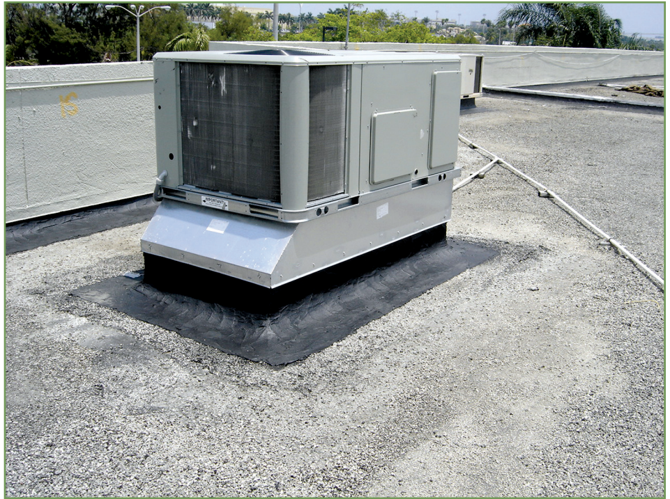
Metal counterflashing over base flashing repair.
