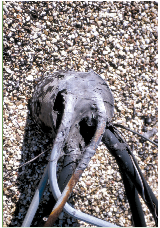
Challenging multiple pipe pitch-pan detail.
