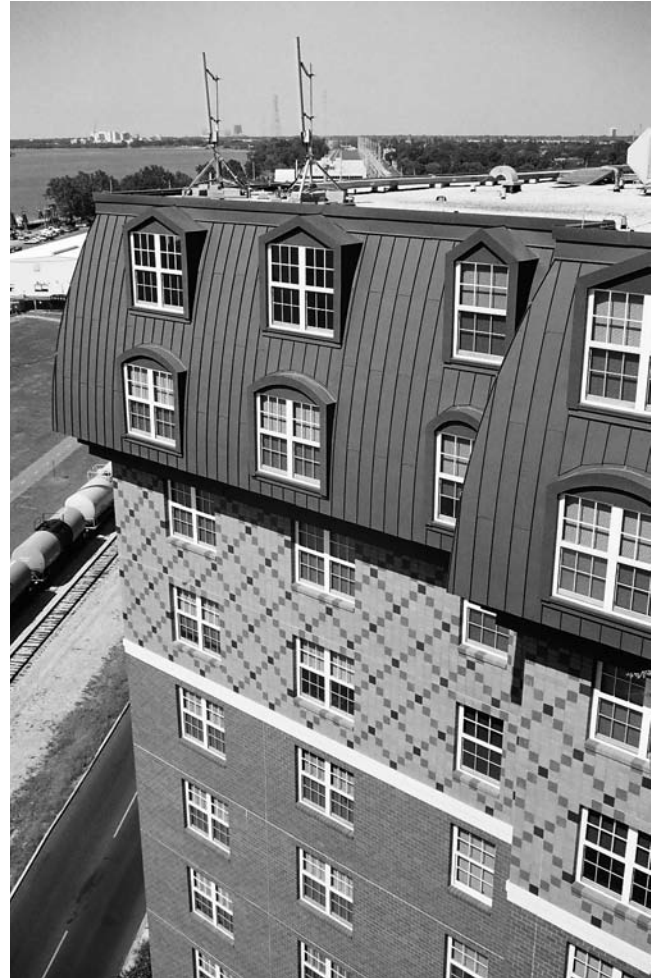
Figure 1 – Typical elevation showing intricate masonry.
