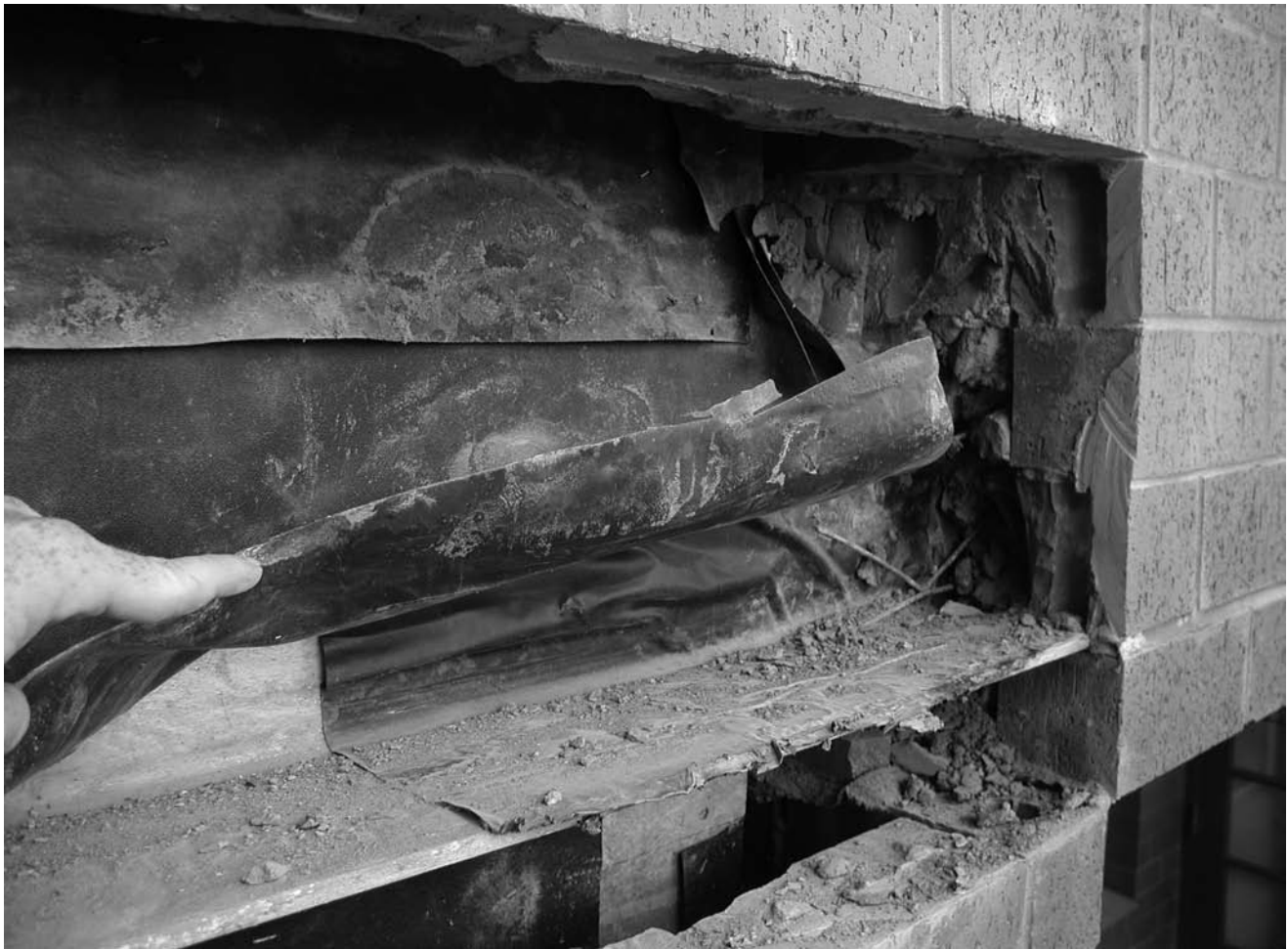
Figure 16 – PVC flashing lap set “dry.”
